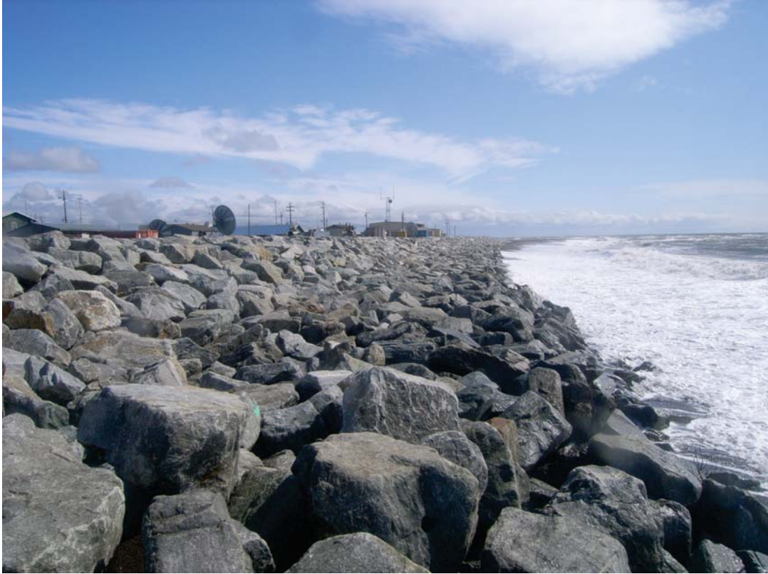
Riprap revetment, July 2011
