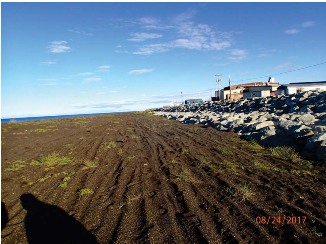
Typical Riprap revetment , August 2017
