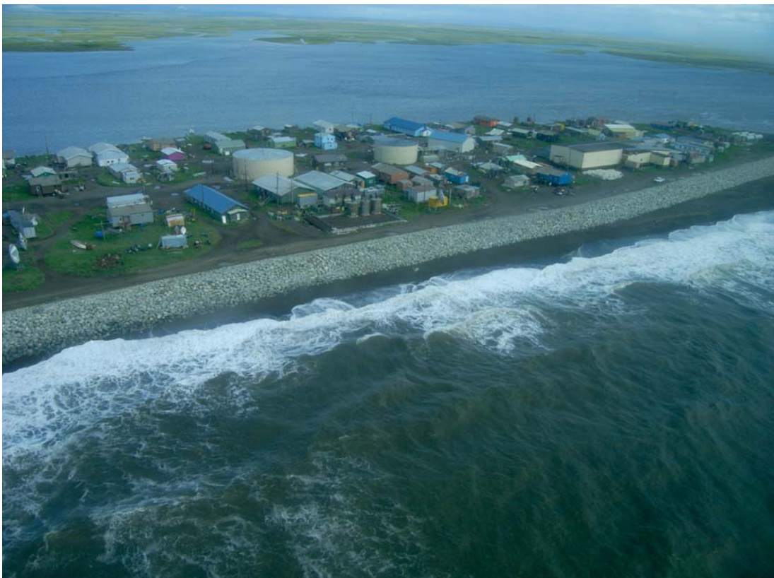
Oblique of the riprap revetment, July 2011
