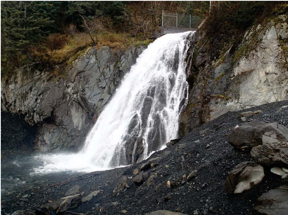
The tunnel outlet, April 2016
