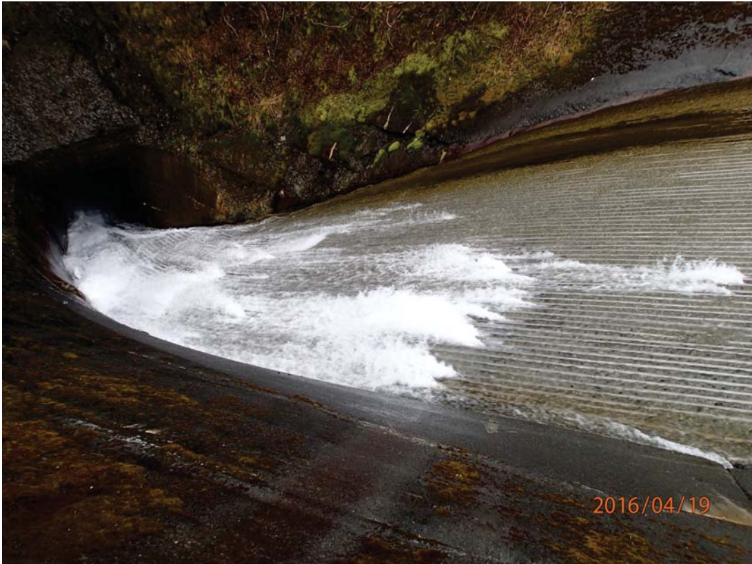
Inlet to the Lowell Creel Tunnel, April 2016
