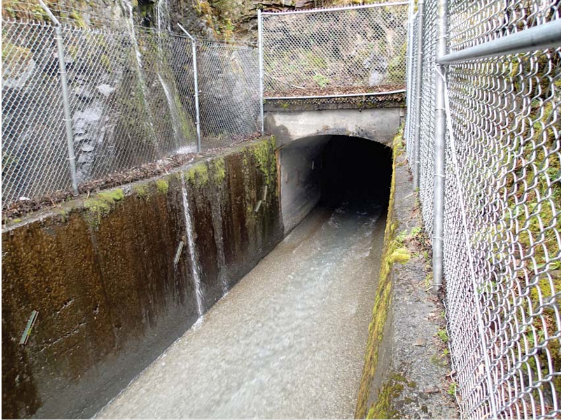
Looking upstream at tunnel outlet, April 2016
