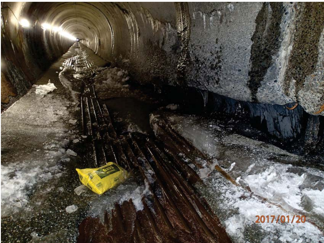
Tunnel damage looking downstream, January 2017
