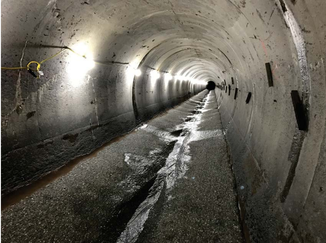
Looking downstream inside tunnel, January 2017
