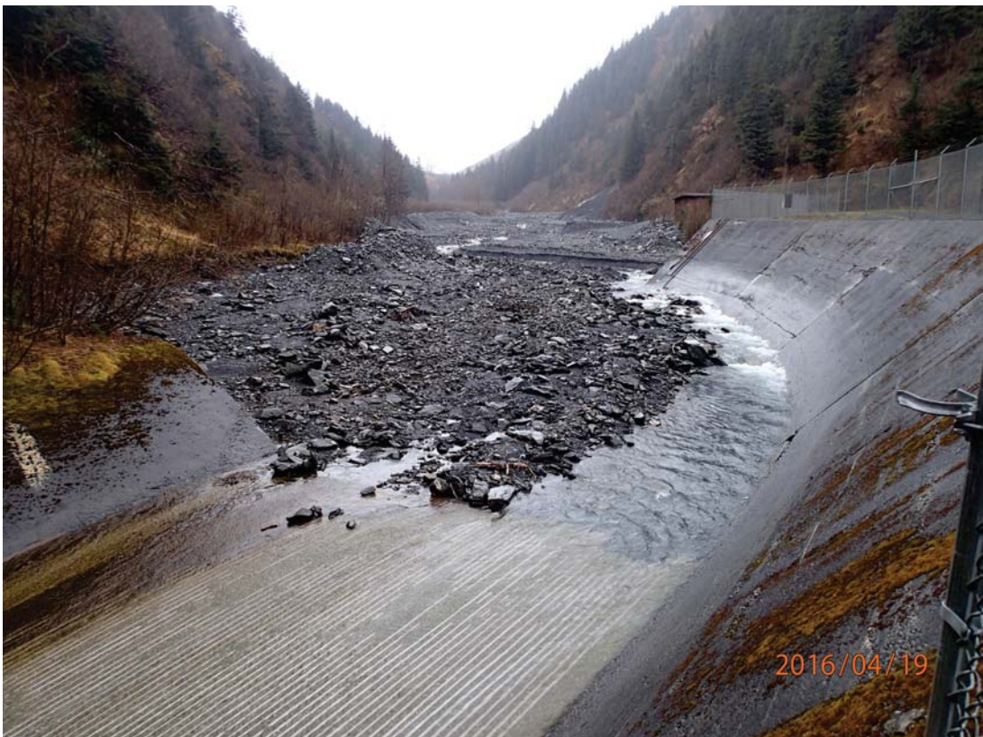
Looking upstream at Lowell Creek and the diversion dam, April 2016
