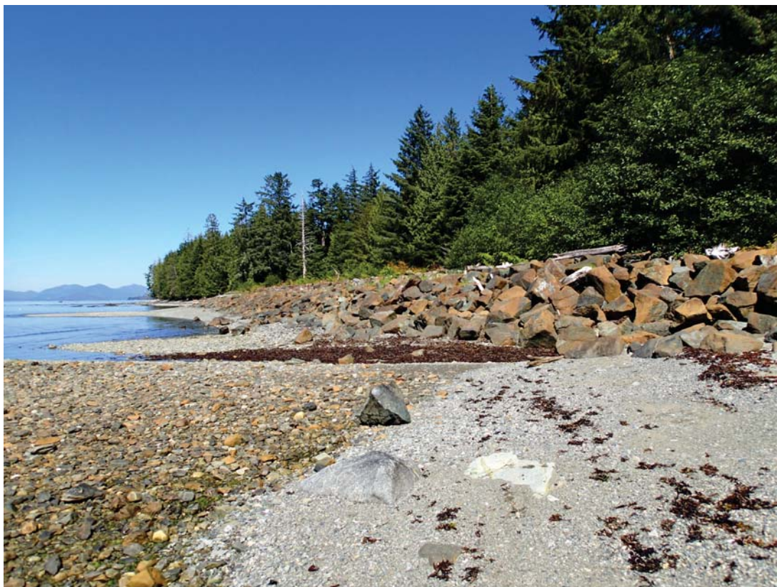
The cemetery rock revetment , August 2017
