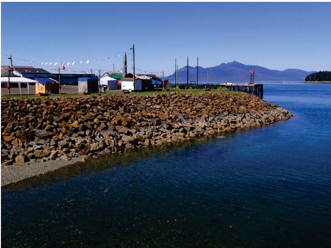
City Park rock revetment, August 2017
