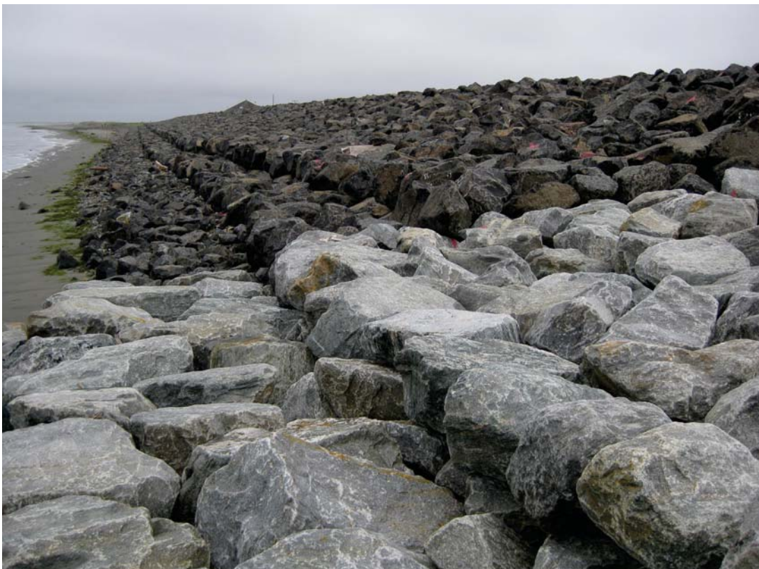
Rock revetment , August 2010
