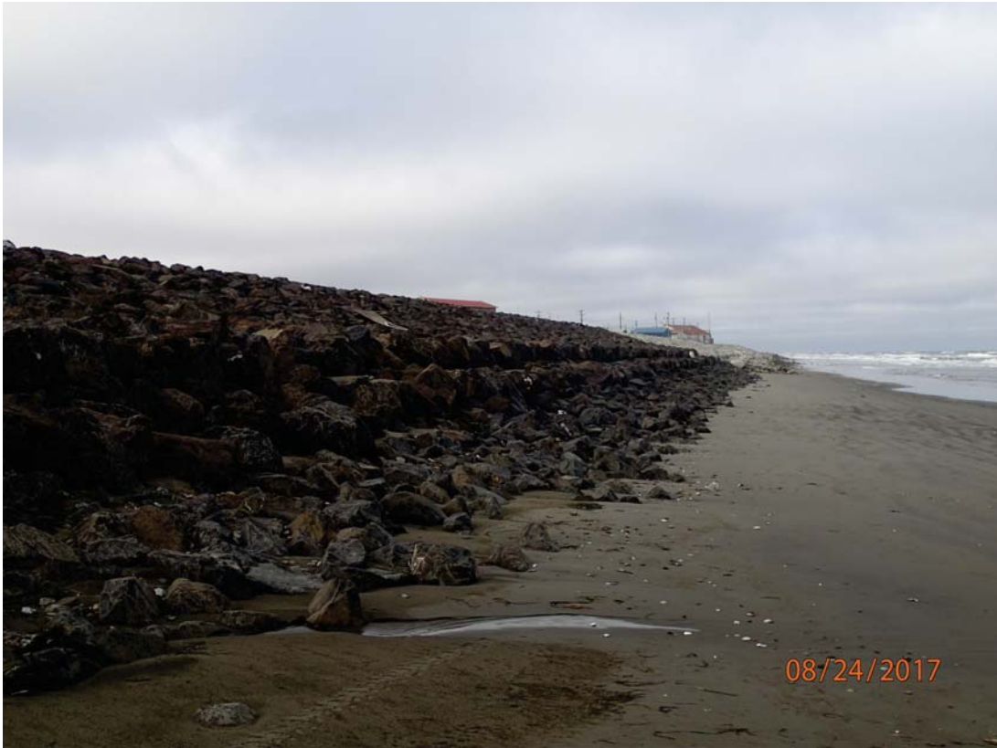
Rock revetment , August 2017
