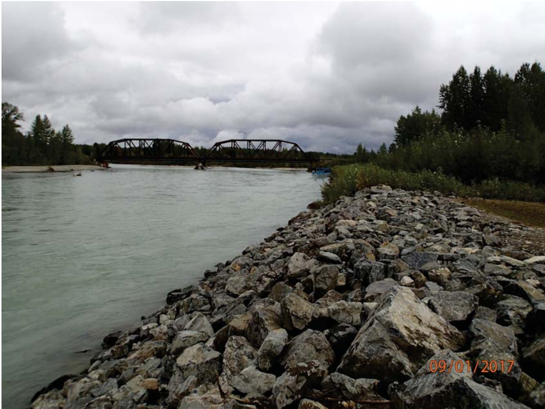
Upstream view of the rock revetment and the railroad bridge, September 2017
