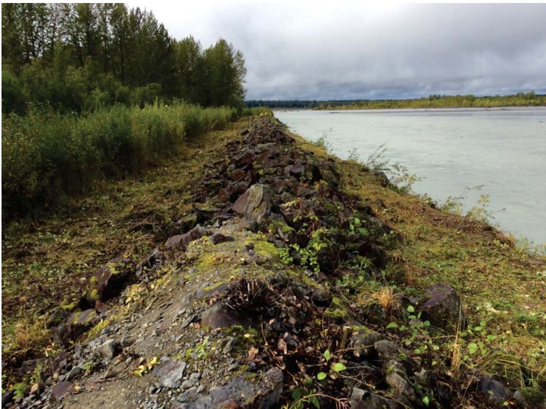
Downstream view of the rock revetment, October 2014
