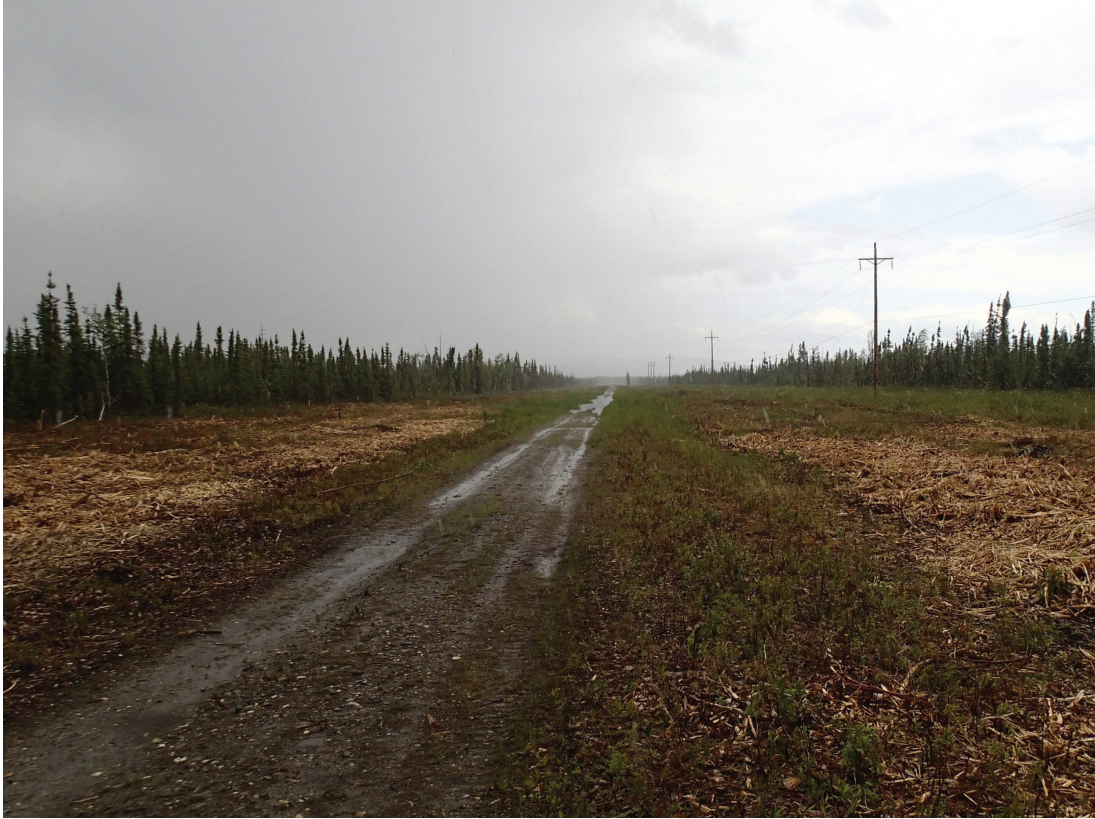
The East Cutoff Dike, June 2014
