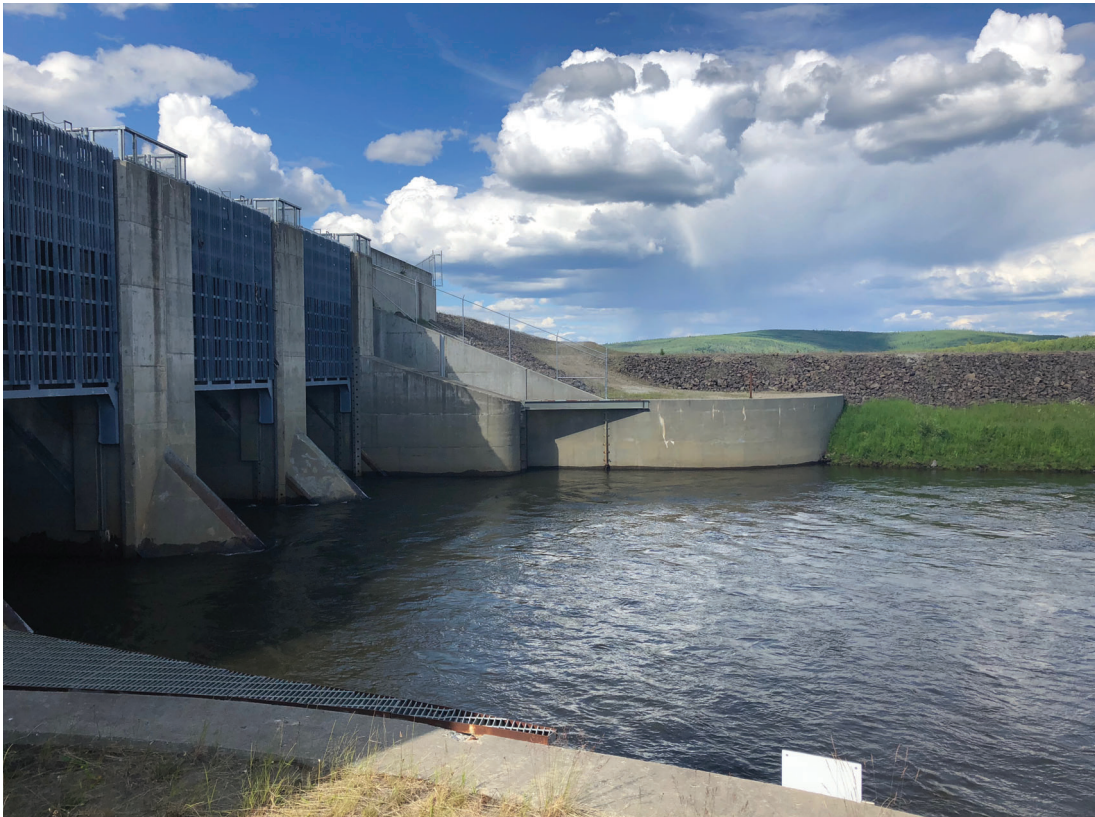
Control Works during inspection, June 2018
