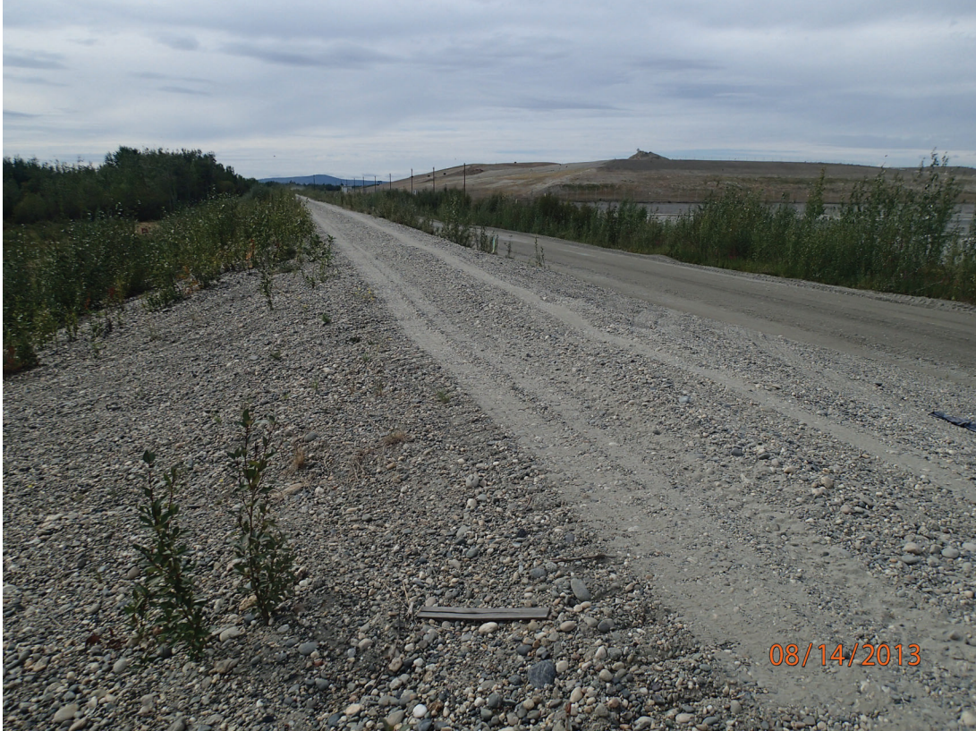
Crest of the Tanana River Levee, August 2013
