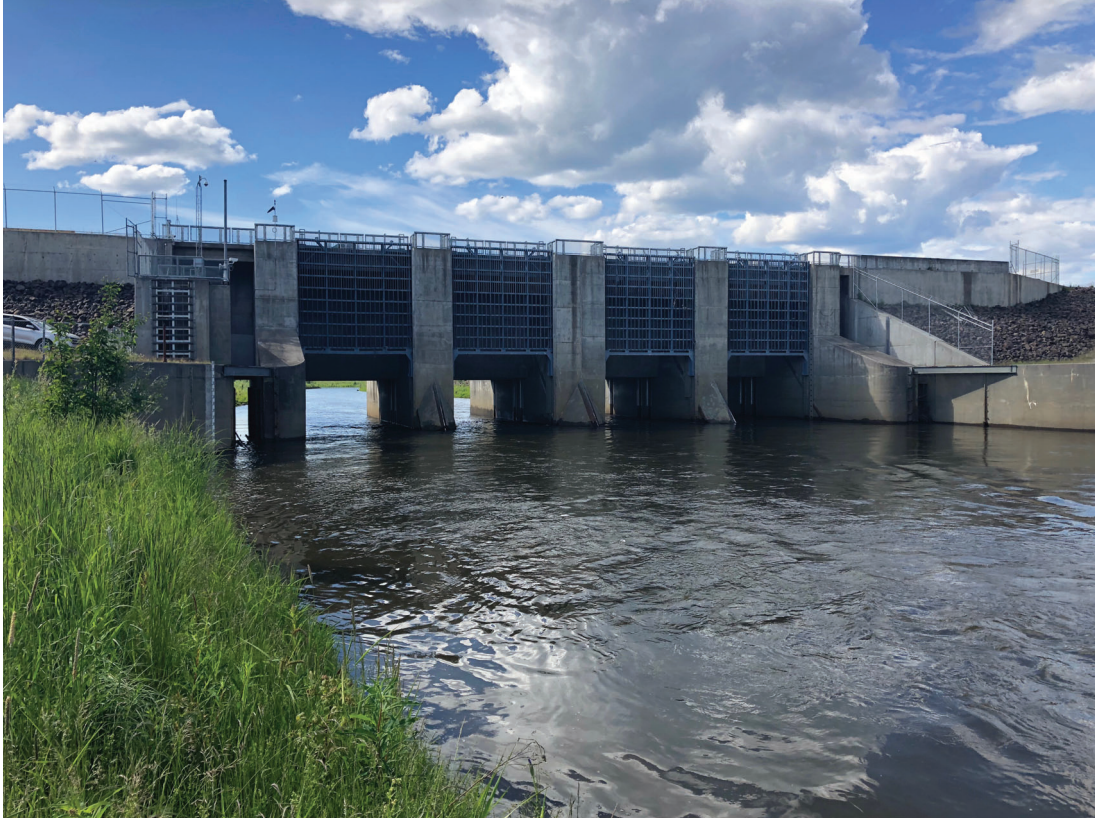
Control Works during inspection, June 2018
