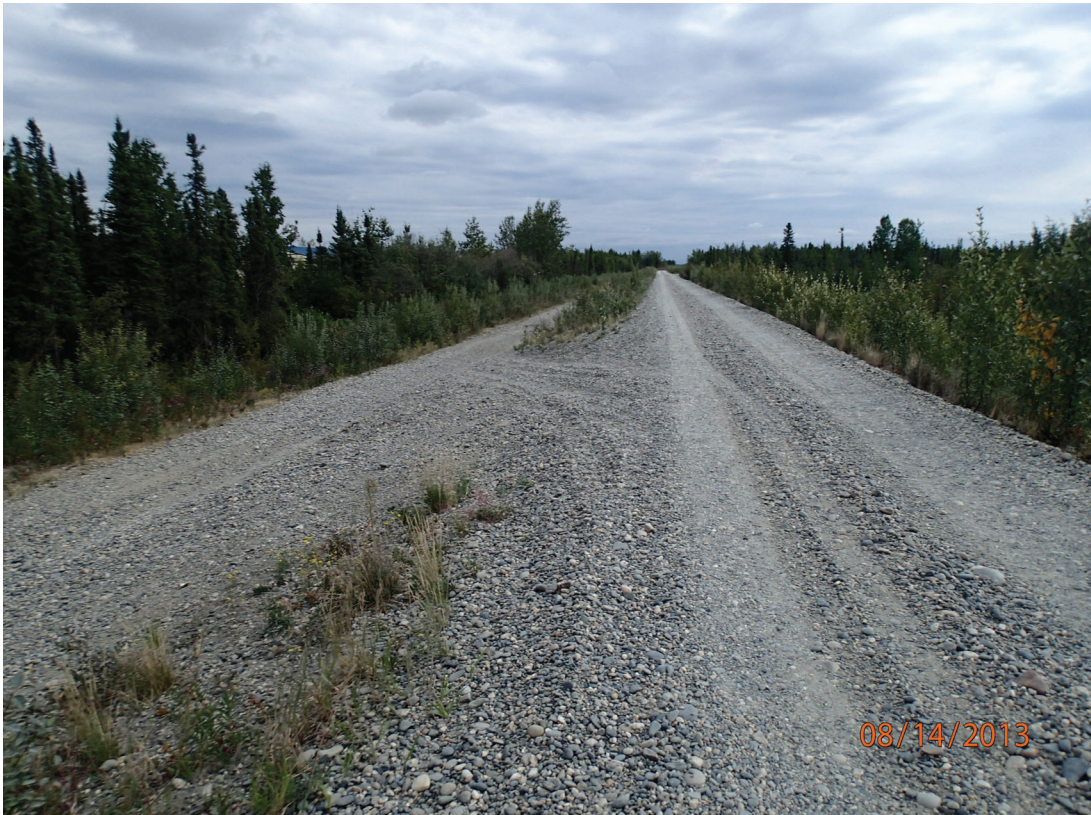
Crest of the Tanana River Levee, August 2013
