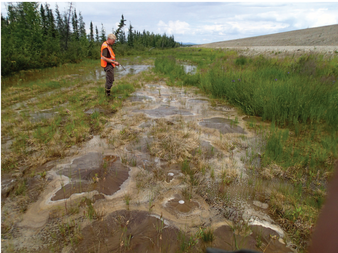
Sand boils in the toe of the stability berm during the 2014 flood event, July 2014
