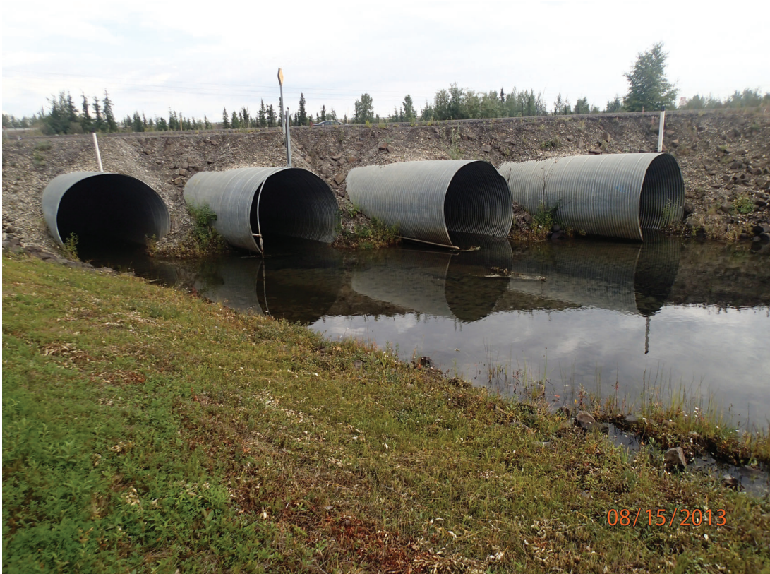
Culverts within the Tanana River Levee, August 2013
