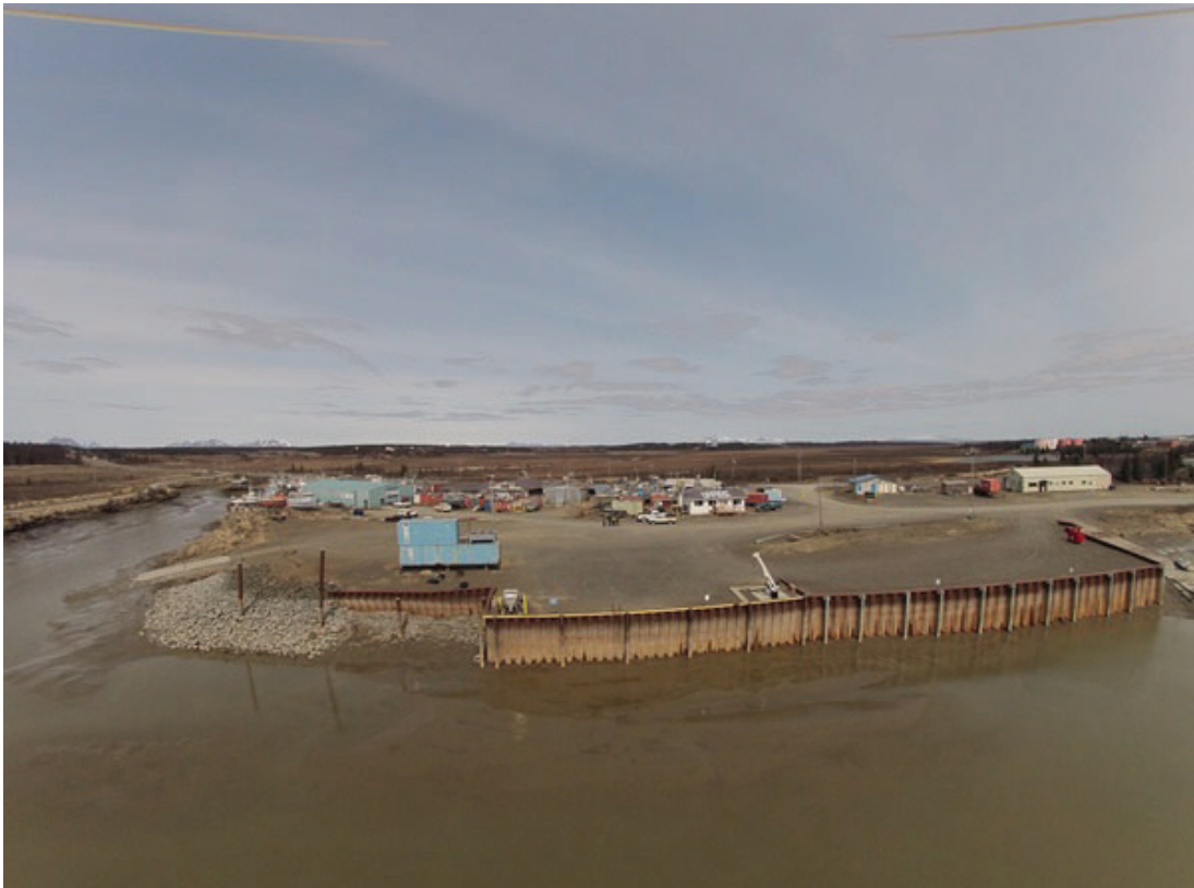
Riprap and sheetpile protection on the east side of the entrance channel, May 2014
