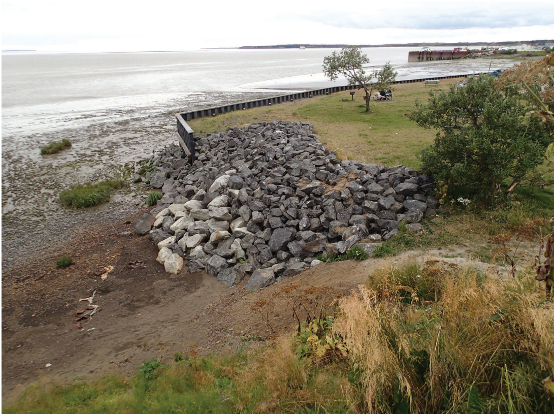
Rip-rap protection at the eastern extent of bank stabilization, August 2019
