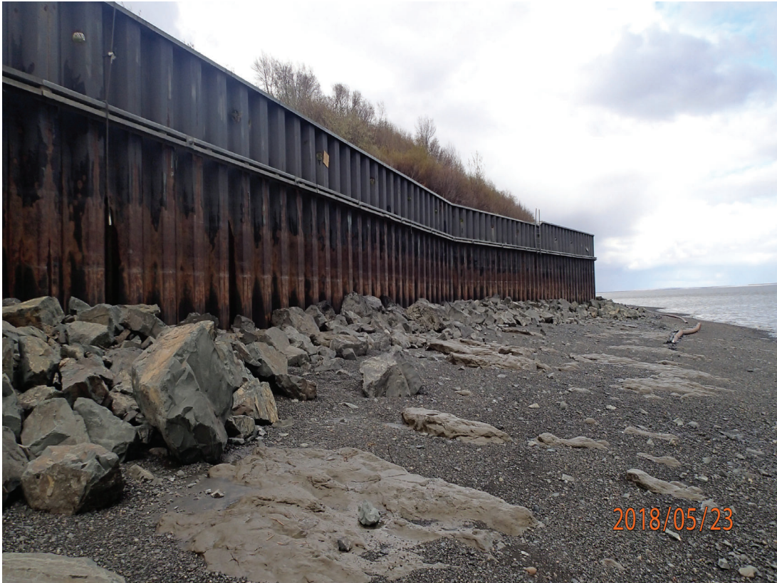
H-pile supported sheetpile bulkhead, May 2018
