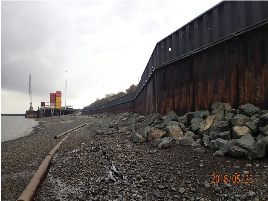
STA 17+00 Riprap @ Toe, Facing Downstream, May 2018
