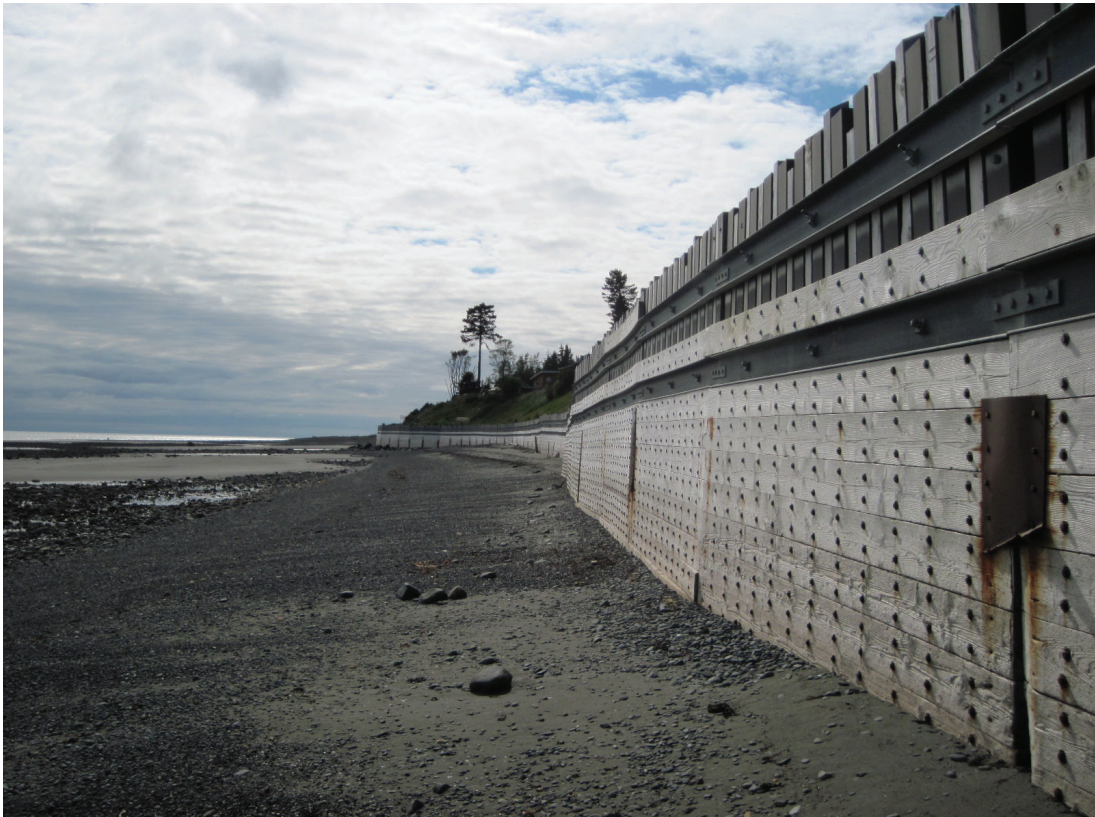
Sheet pile wall at the base of the Homer Spit, June 2011
