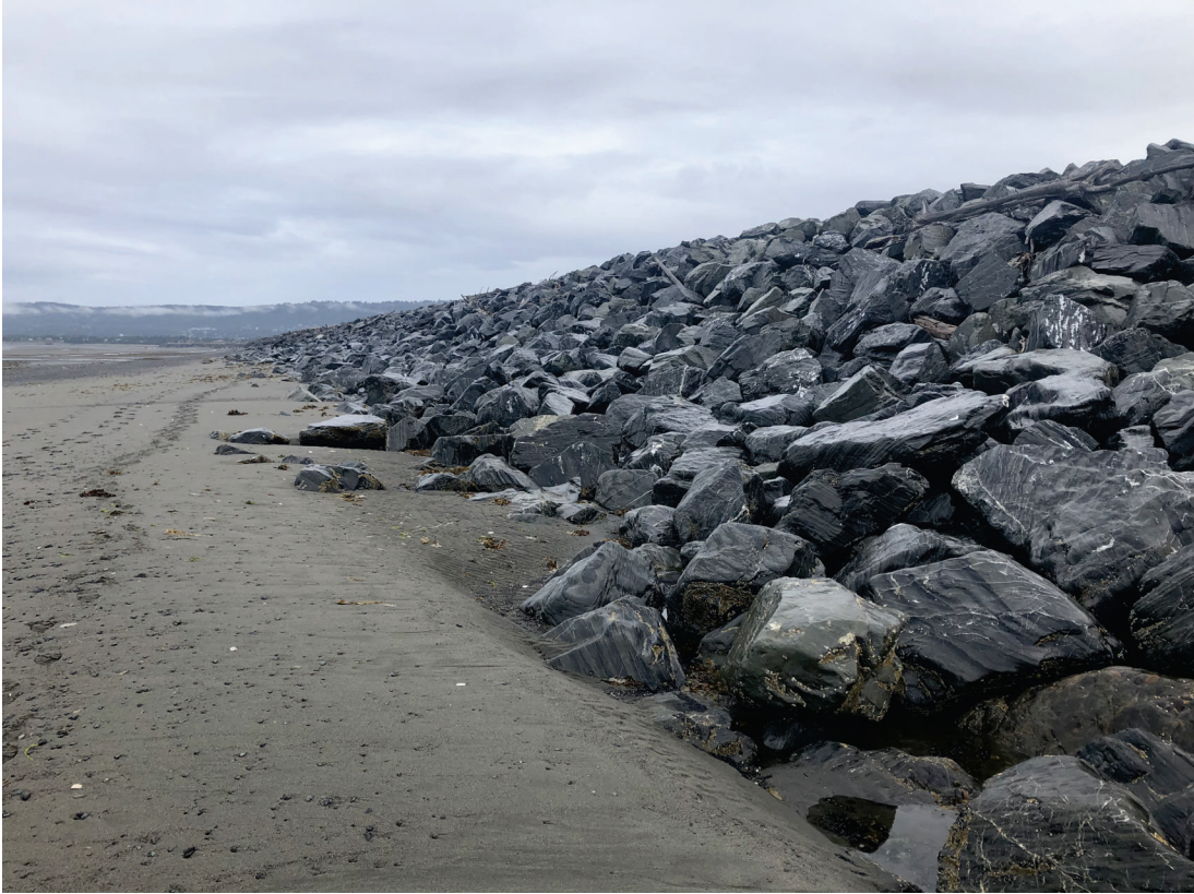
Rock revetment along the Homer Spit, July 2019
