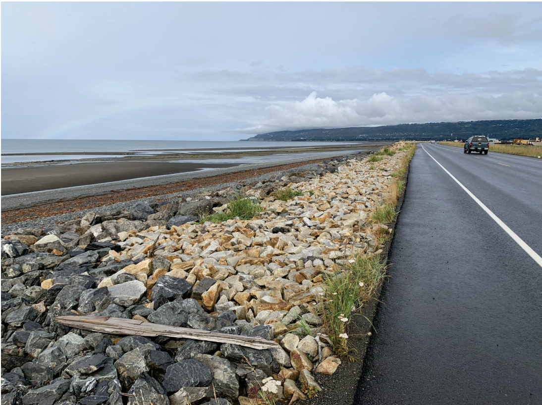
Rock revetment along the Homer Spit, July 2019
