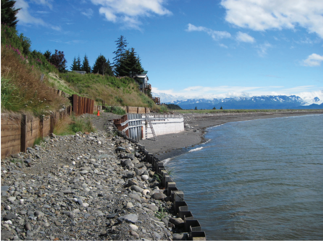
Sheet pile wall at the base of the Homer Spit, August 2010
