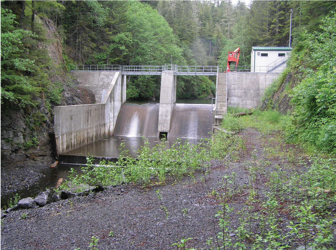
Downstream of Kake Dam, June 2010
