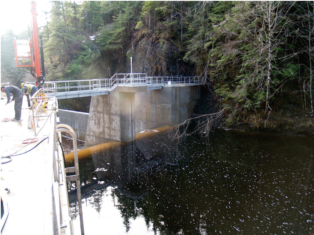
Upstream of Kake Dam during construction, January 2007
