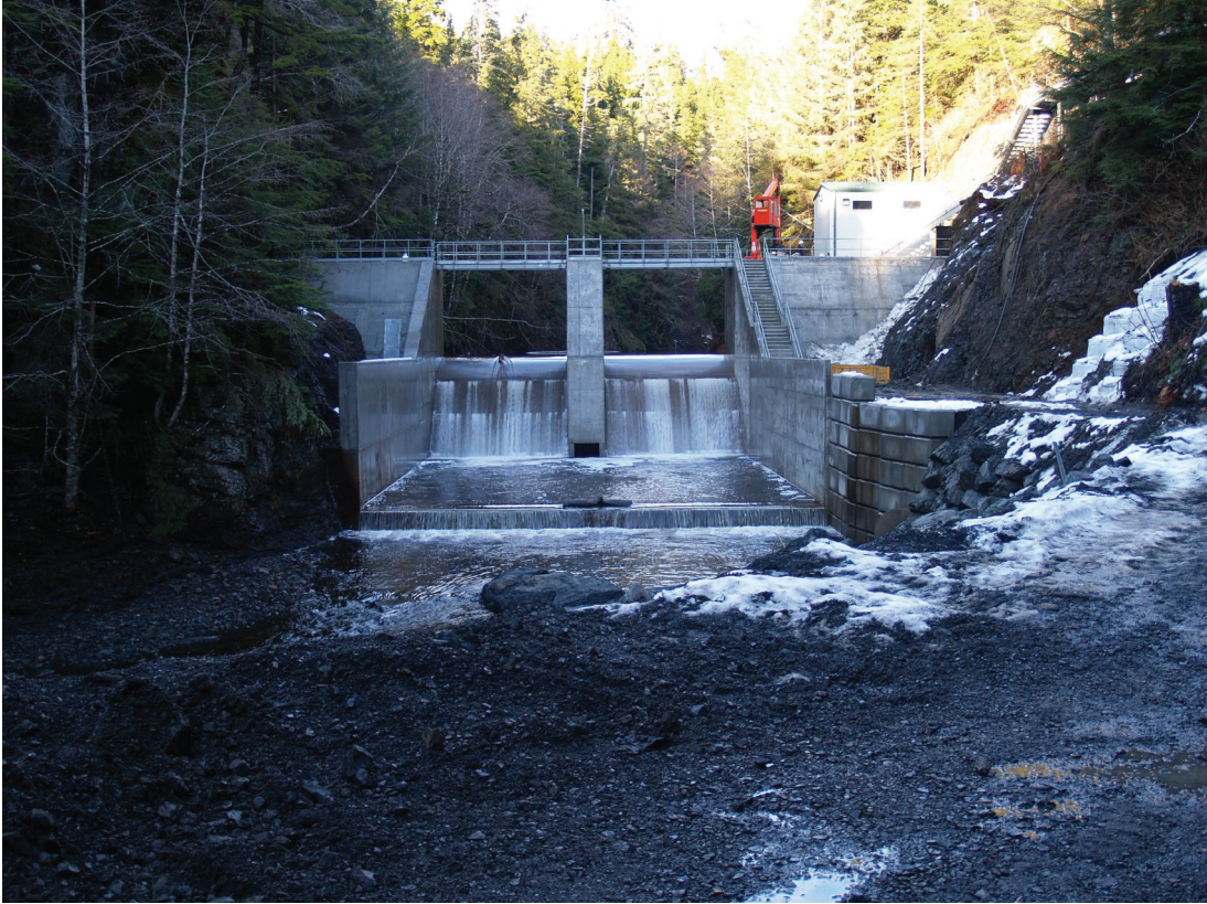
Downstream of Kake Dam during construction, January 2007
