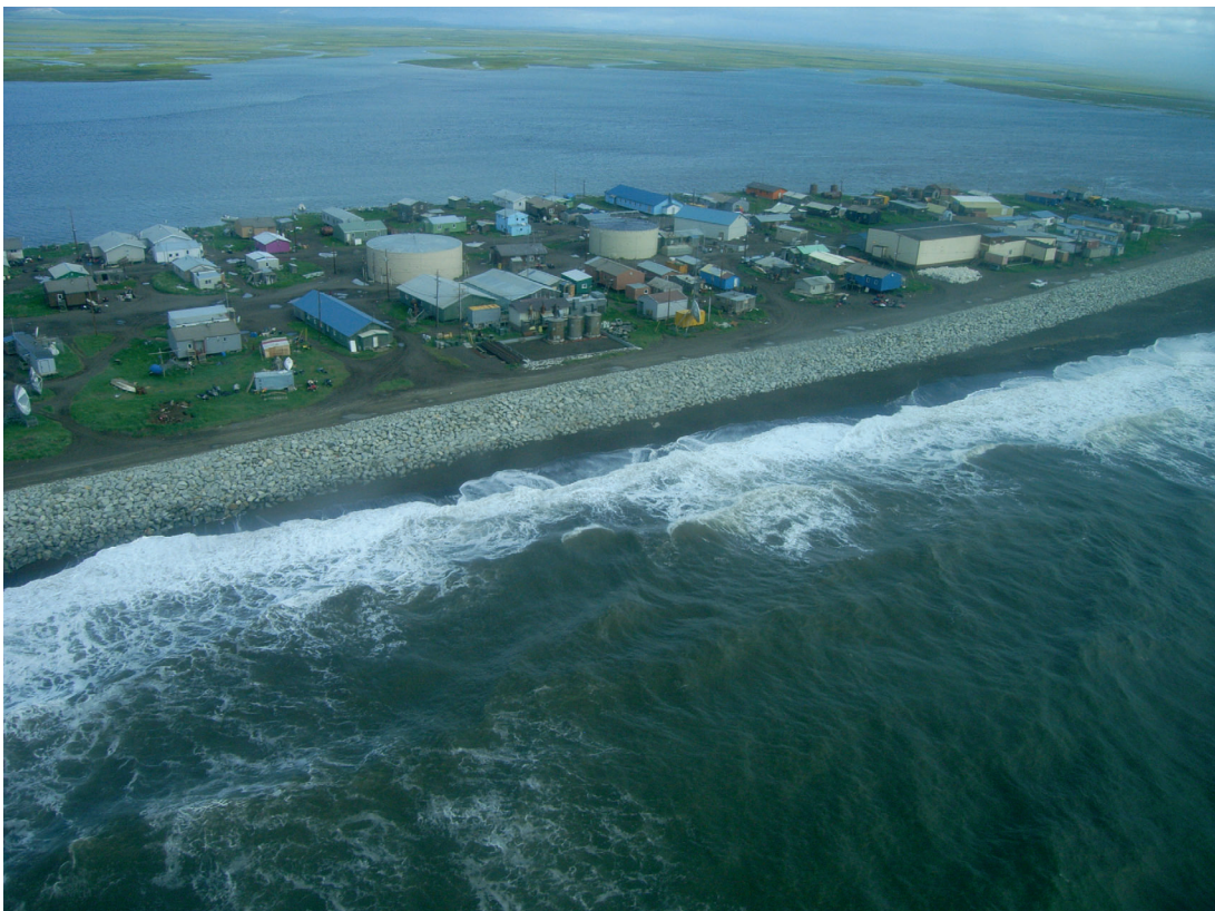
Oblique of the riprap revetment, July 2011
