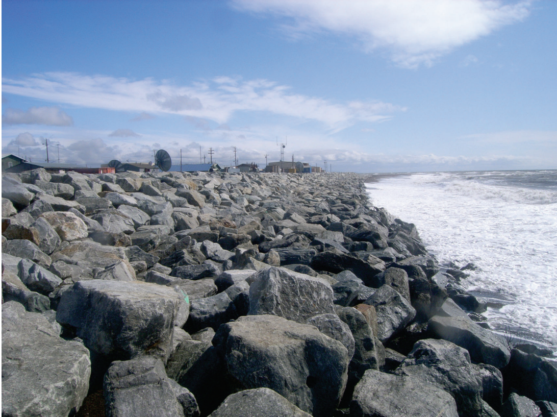
Riprap revetment, July 2011
