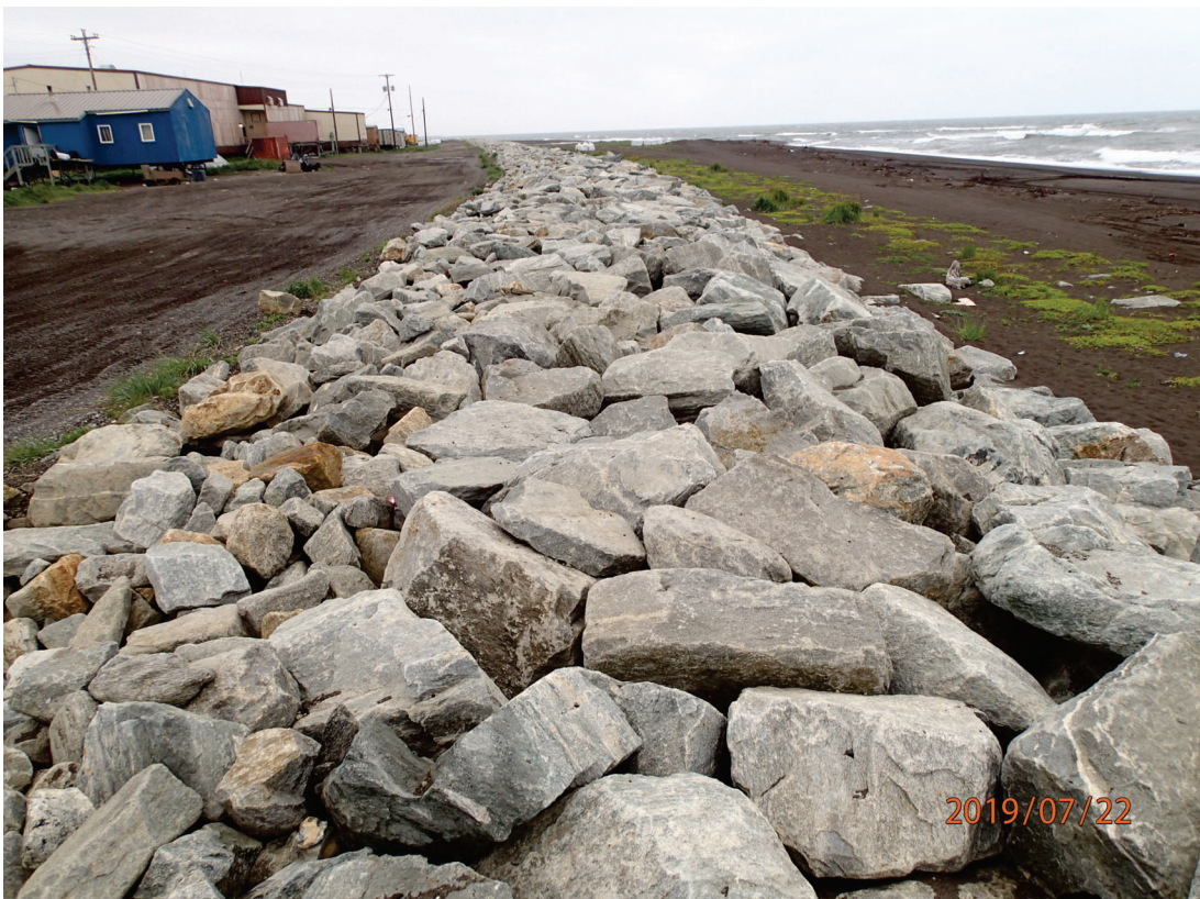
Typical Riprap revetment , July 2019
