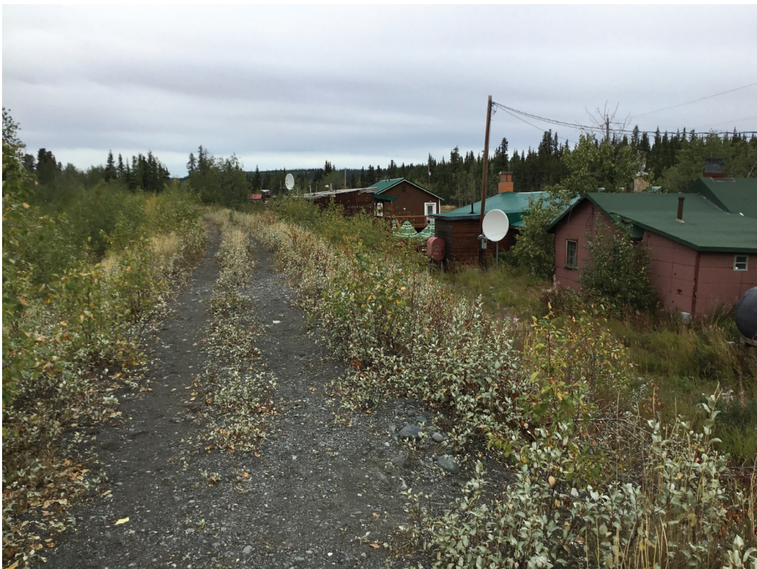
Encroachments within the levee footprint, August 2017
