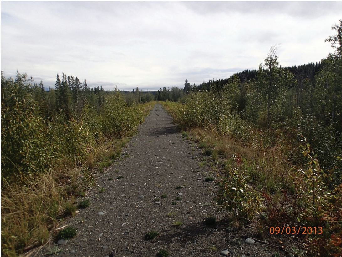
Klutina River Levee, September 2013
