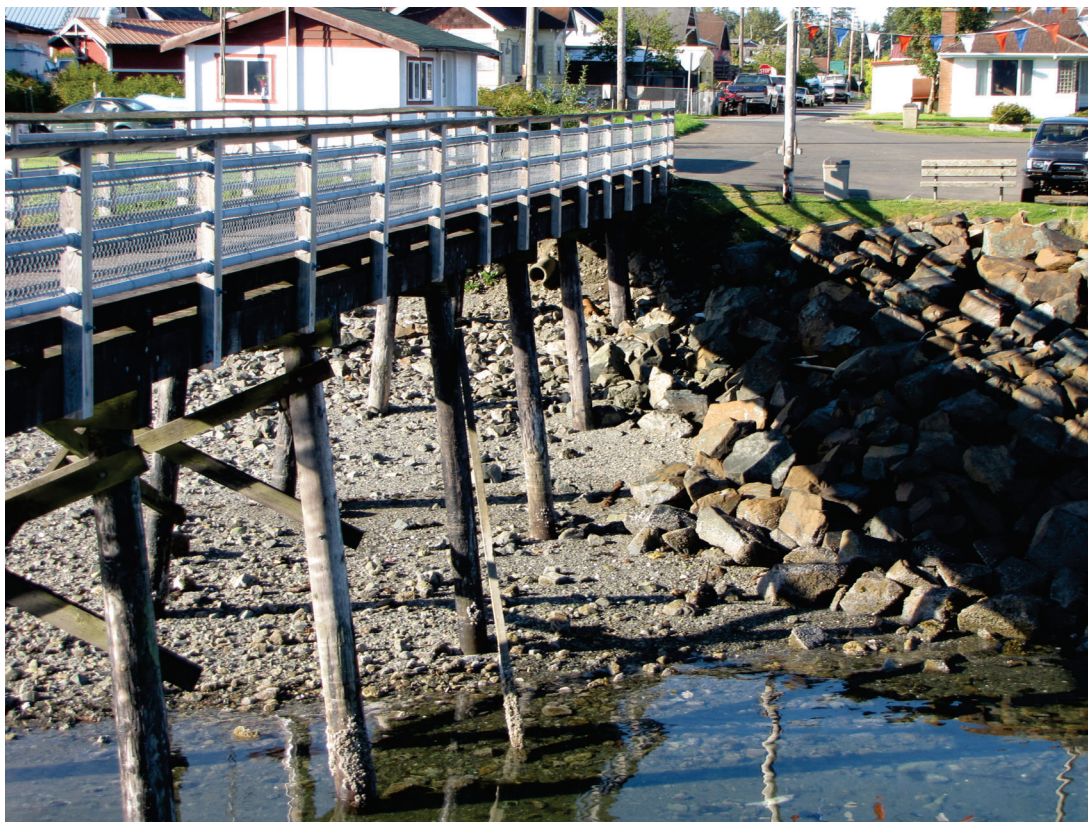
The east extent of the tank farm rock revetment , September 2010
