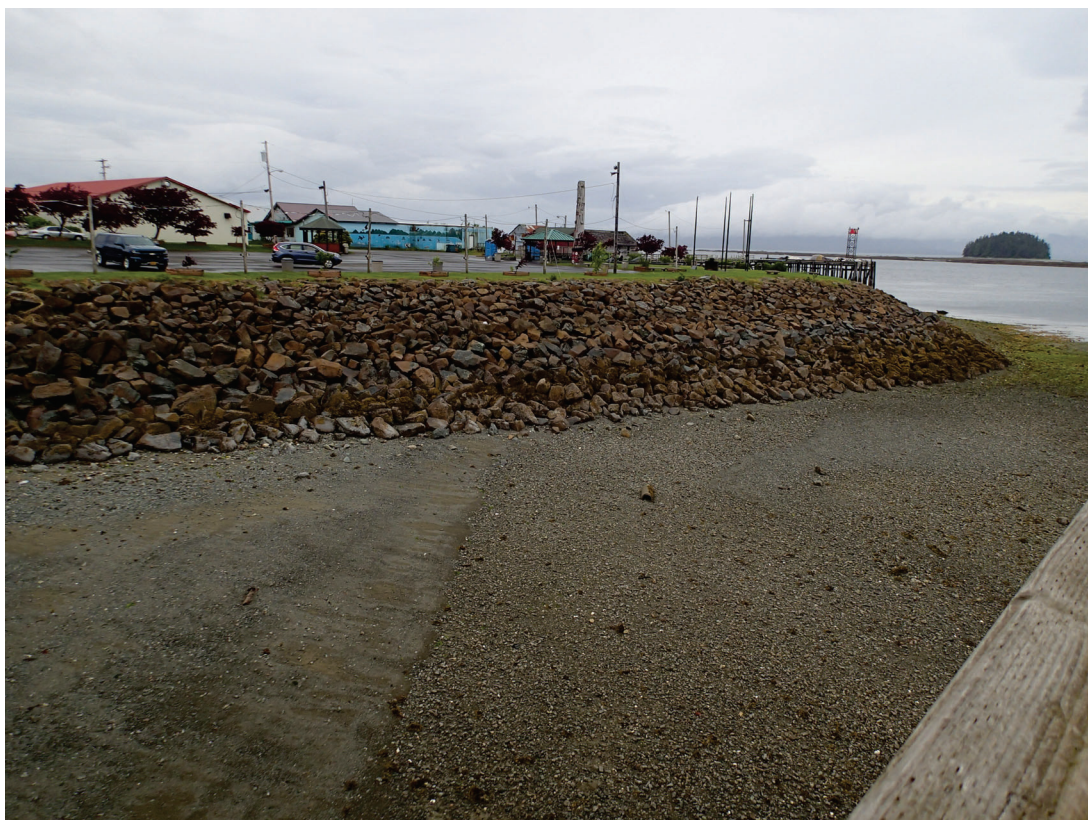
City Park rock revetment, June 2019
