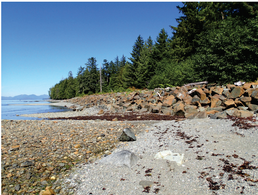
The cemetery rock revetment , August 2017
