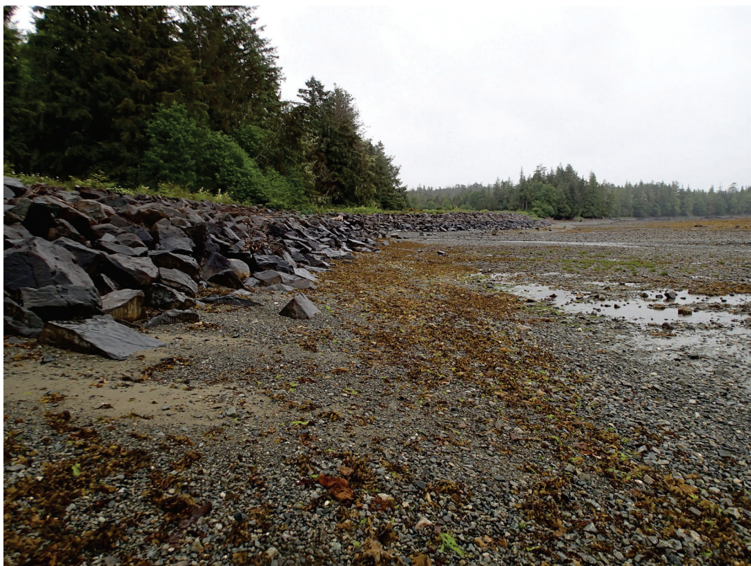
The cemetery rock revetment , June 2019
