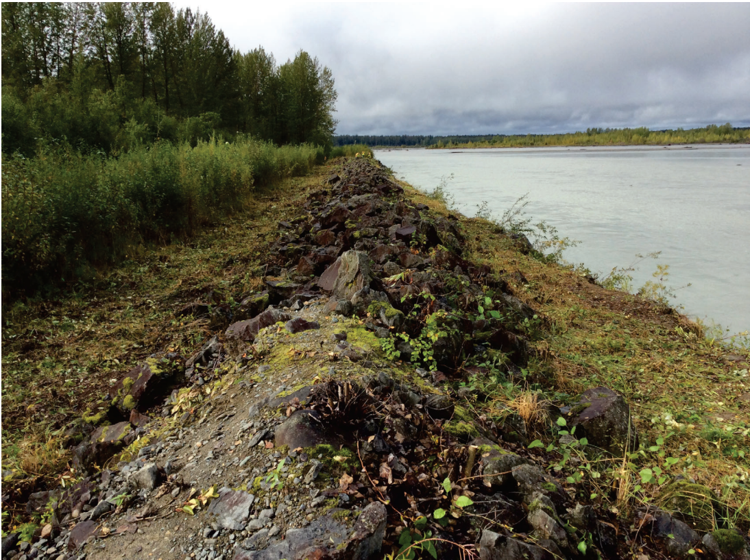
Downstream view of the rock revetment, October 2014
