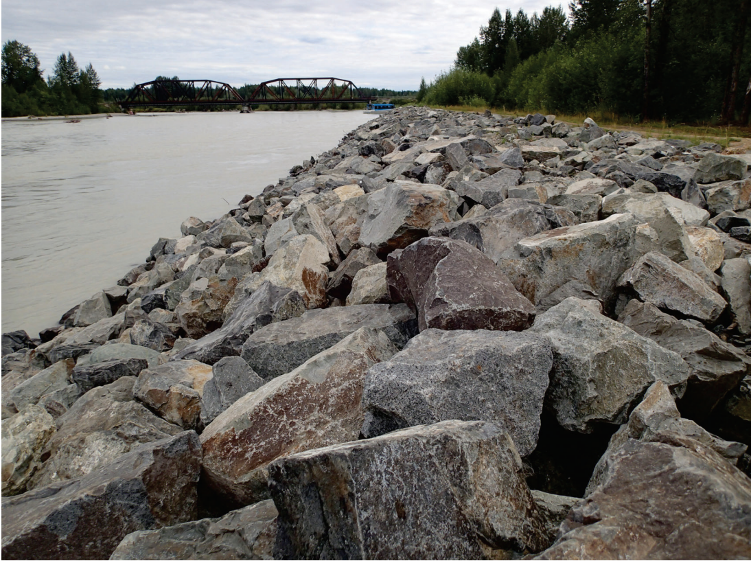
Upstream view of the rock revetment and the railroad bridge, August 2019
