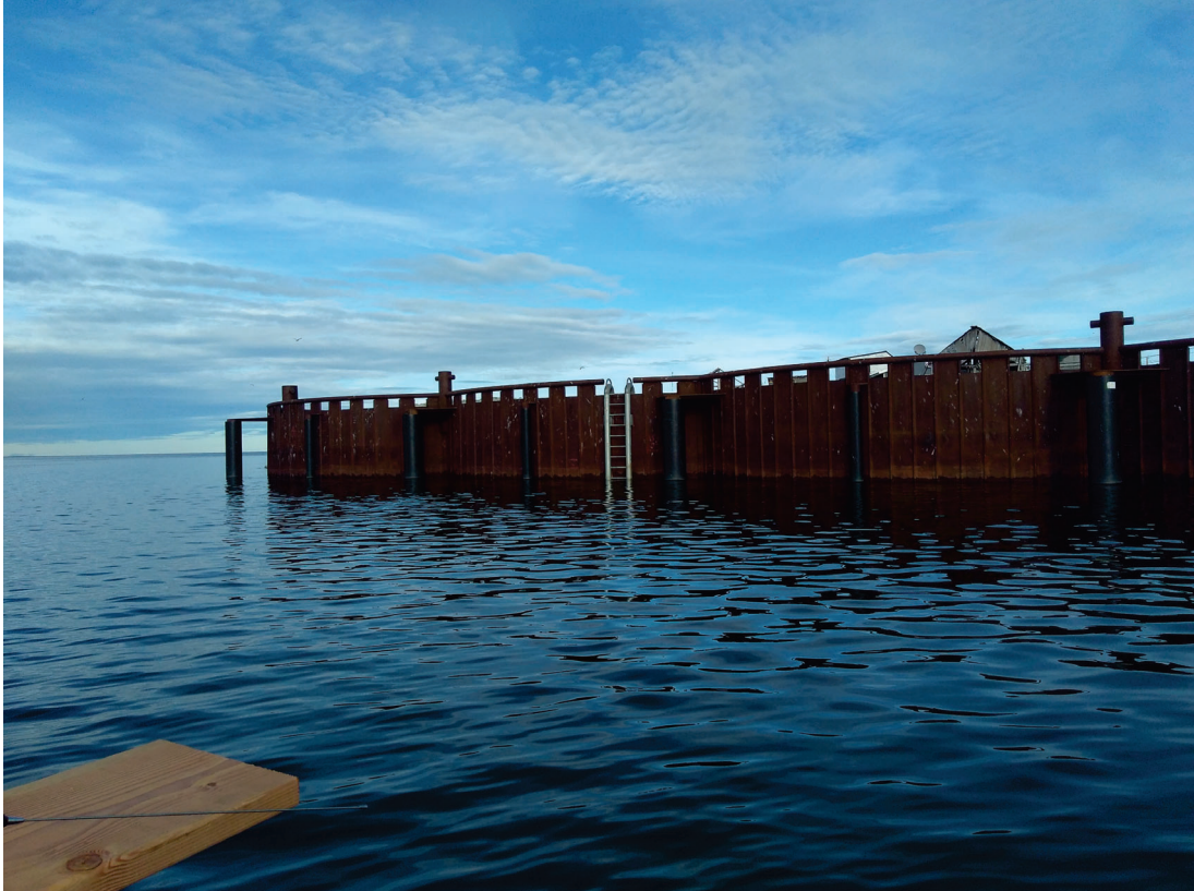
Sheetpile Cells, June 2018
