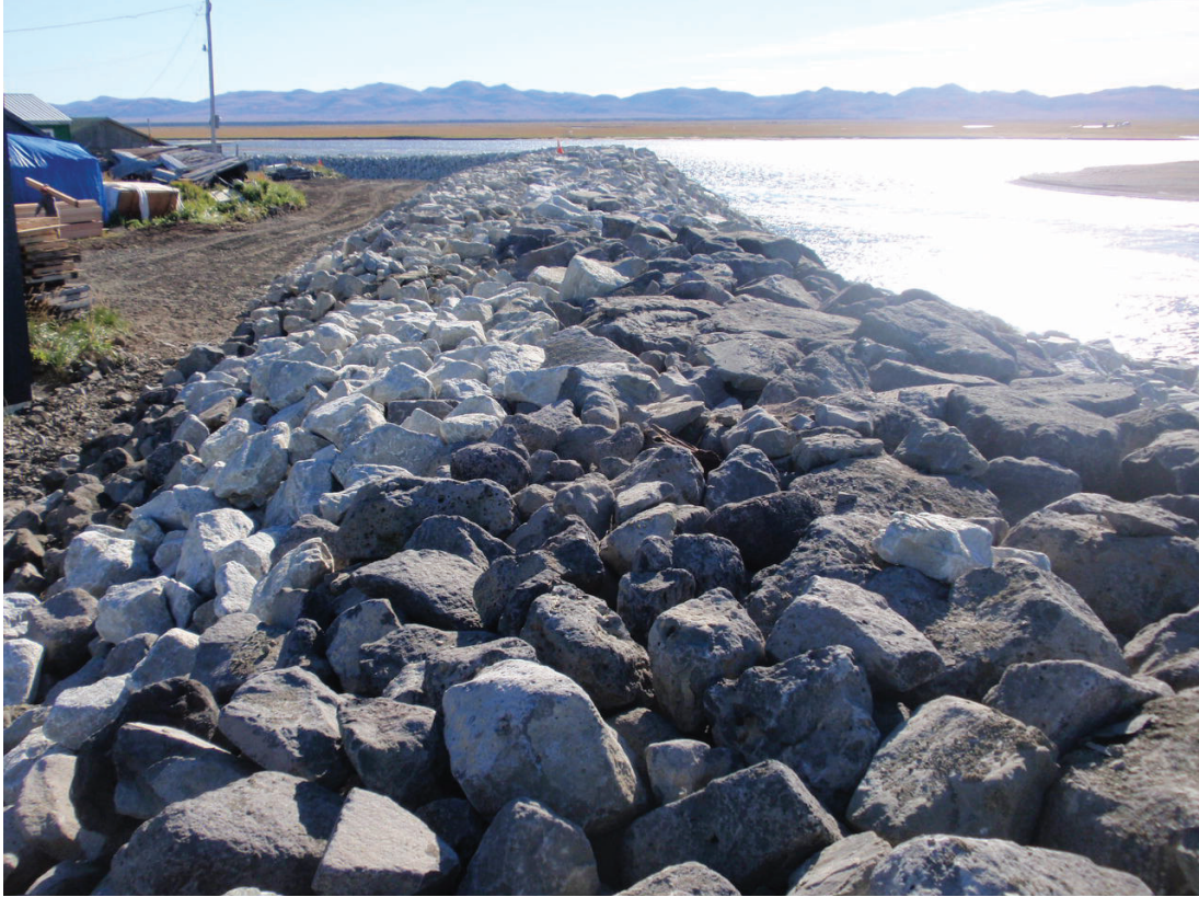
Tie-in to Phase I Project, September 2014
