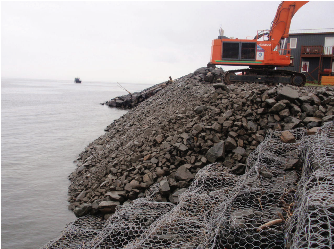
Core rock placed over existing gabions during Phase II, July 2014
