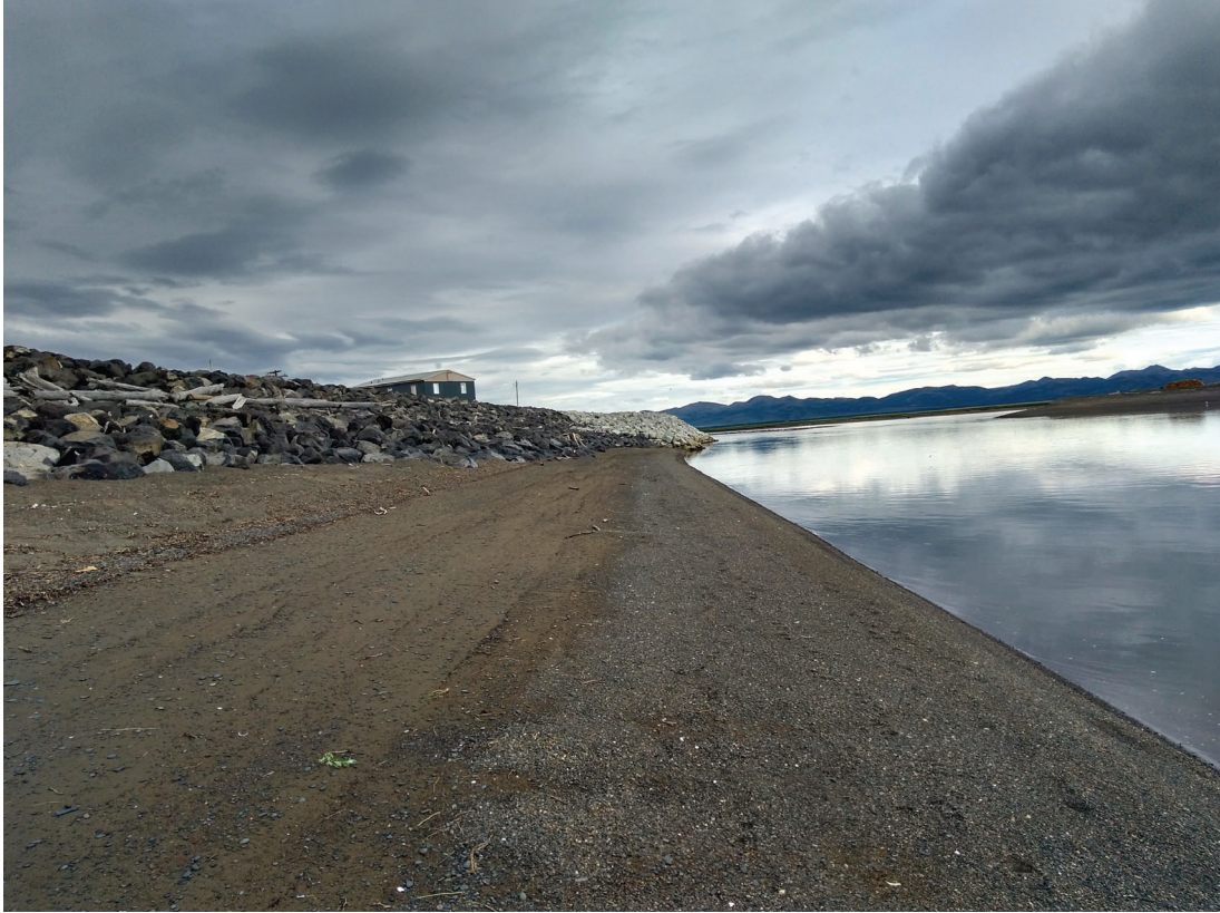
Phase I and Phase II revetments, June 2018
