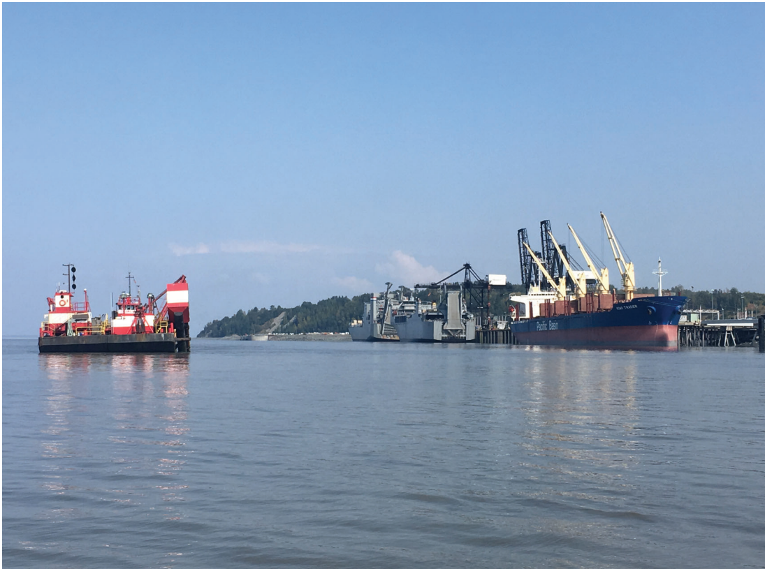
Westport Dredging, August 2019
