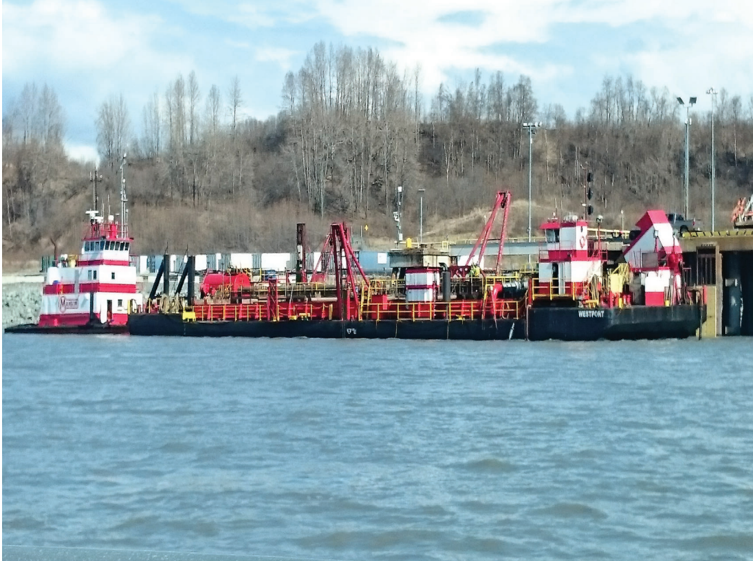
Westport Dredging in Terminal 3, May 2015
