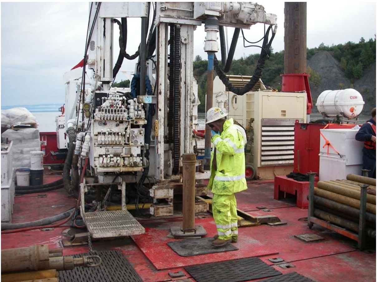
Installing Casing for AP-4629
