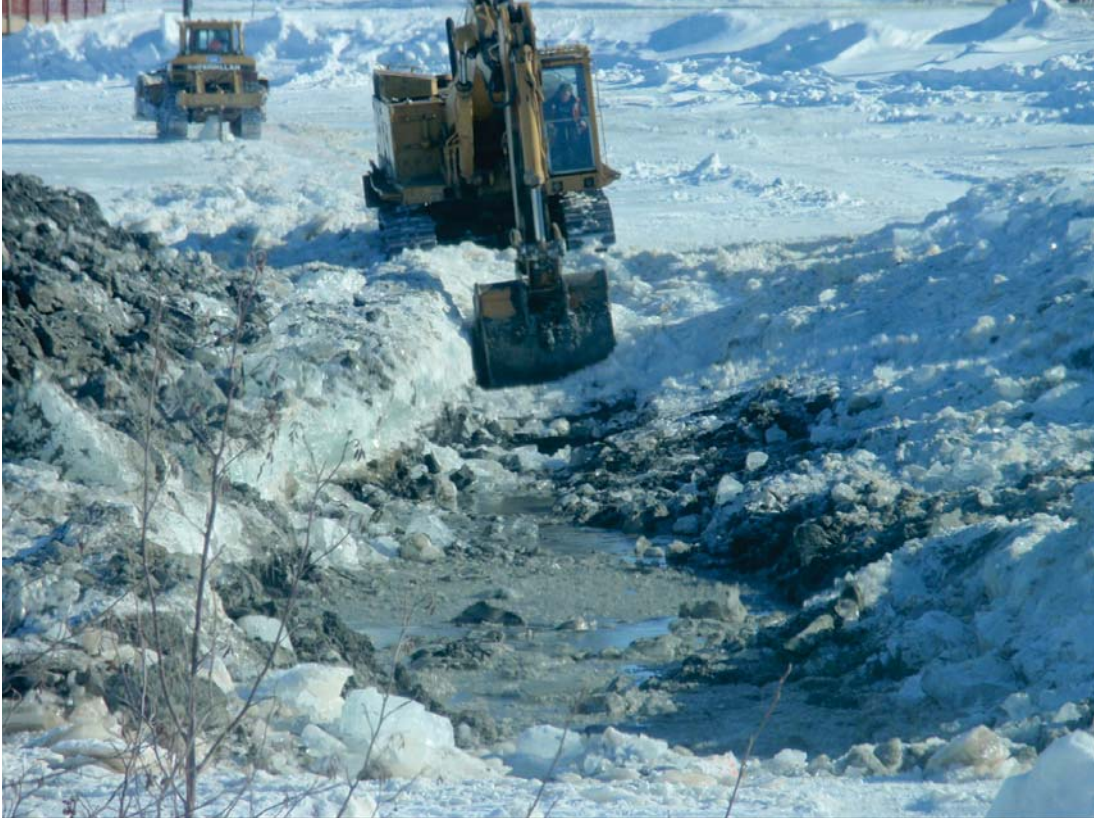
Maintenance dredging of the basin and channel in the winter of 2013.
