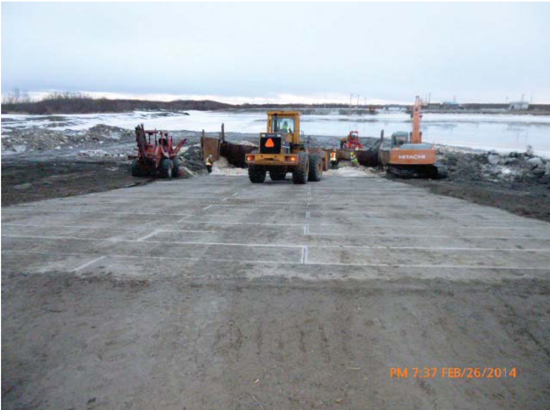
Replacement of the South Ramp, February 2014
