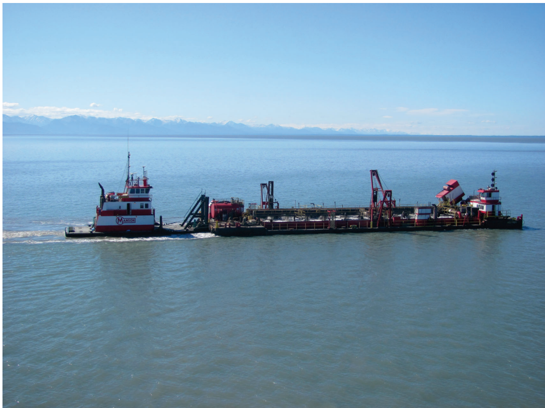
Dredging by Manson's Westport hopper dredge, June 2014
