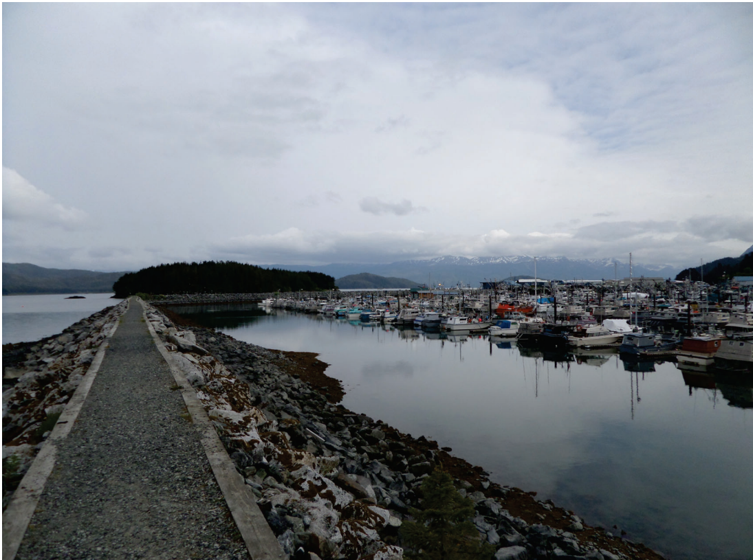
Condition of the western breakwater during May, 2014
