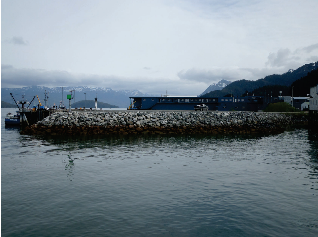
View of the entrance breakwater extension in May, 2014
