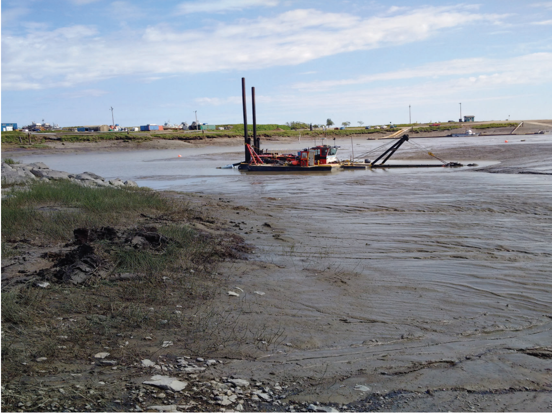
View of maintenance dredging from Scandinavian Creek, May 2016
