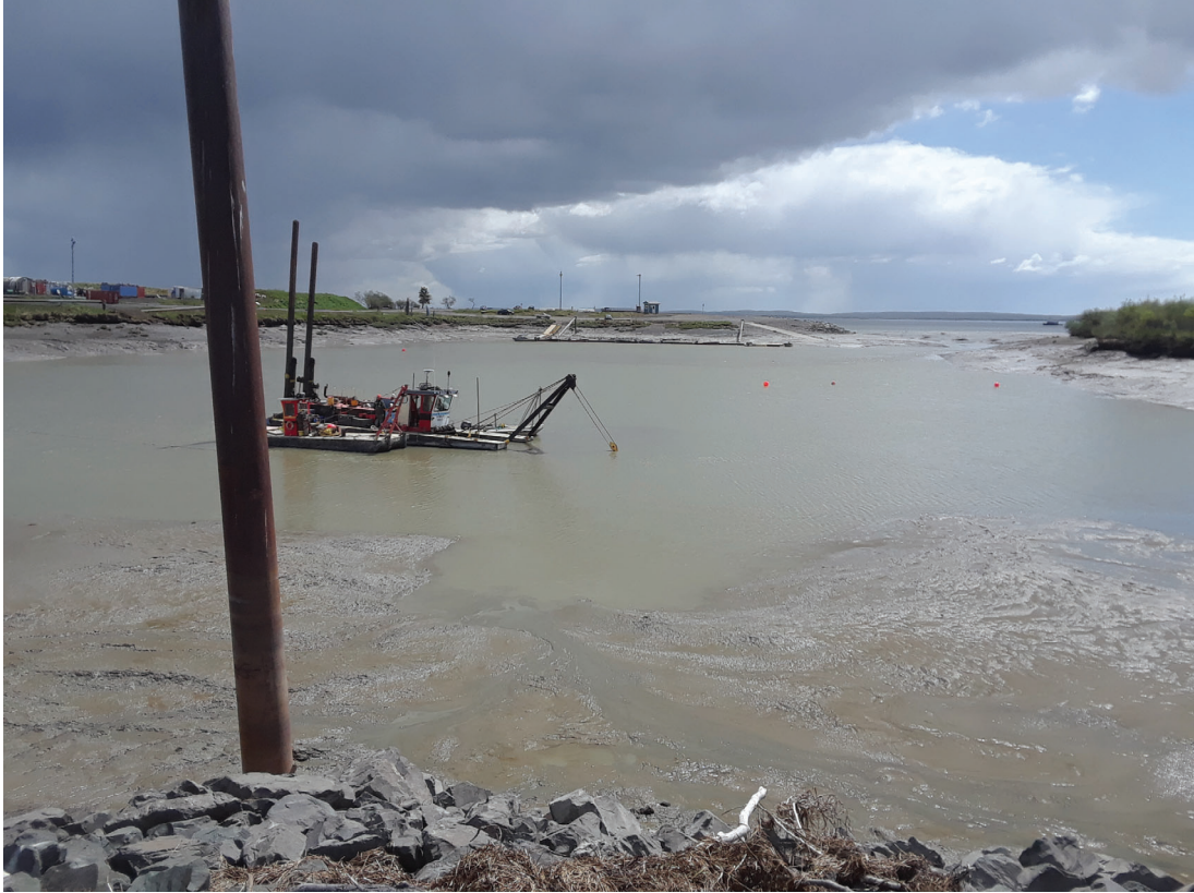
Maintenance dredging of harbor basin, June 2018
