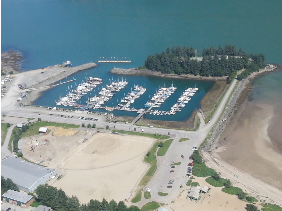
Oblique of Douglas Harbor, July 2013
