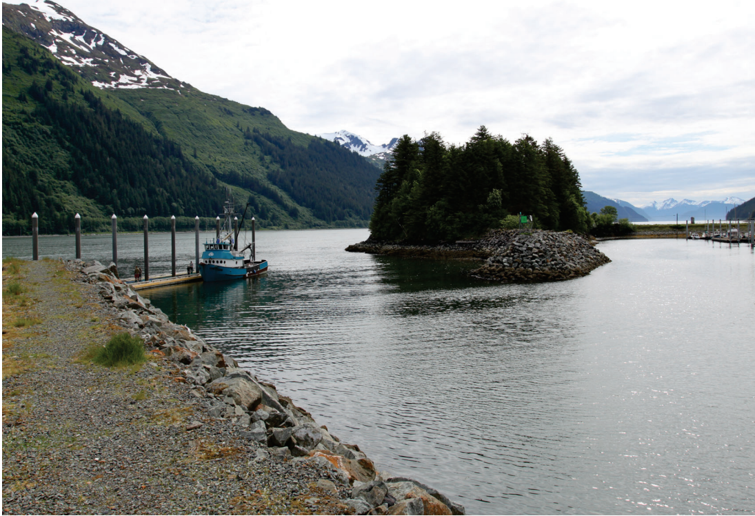
Entrance Channel, June 2017
