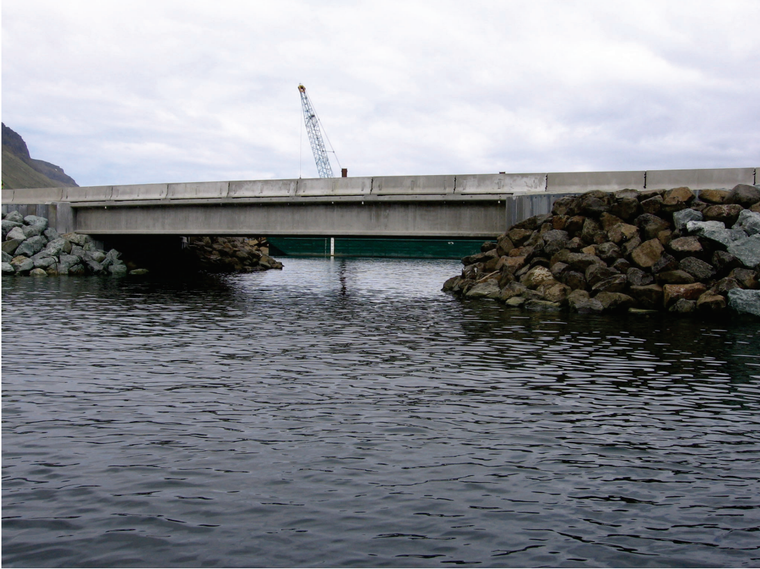
False Pass Harbor Bridge, June 2009
