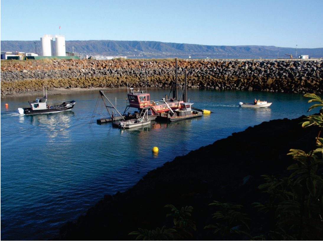
Maintenance dredging of the outer entrance channel, September 2019
