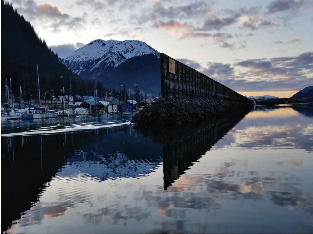
The North end of breakwater at Aurora Harbor, March 2019
