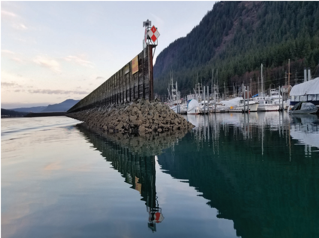
The South end of breakwater at Aurora Harbor, March 2019
