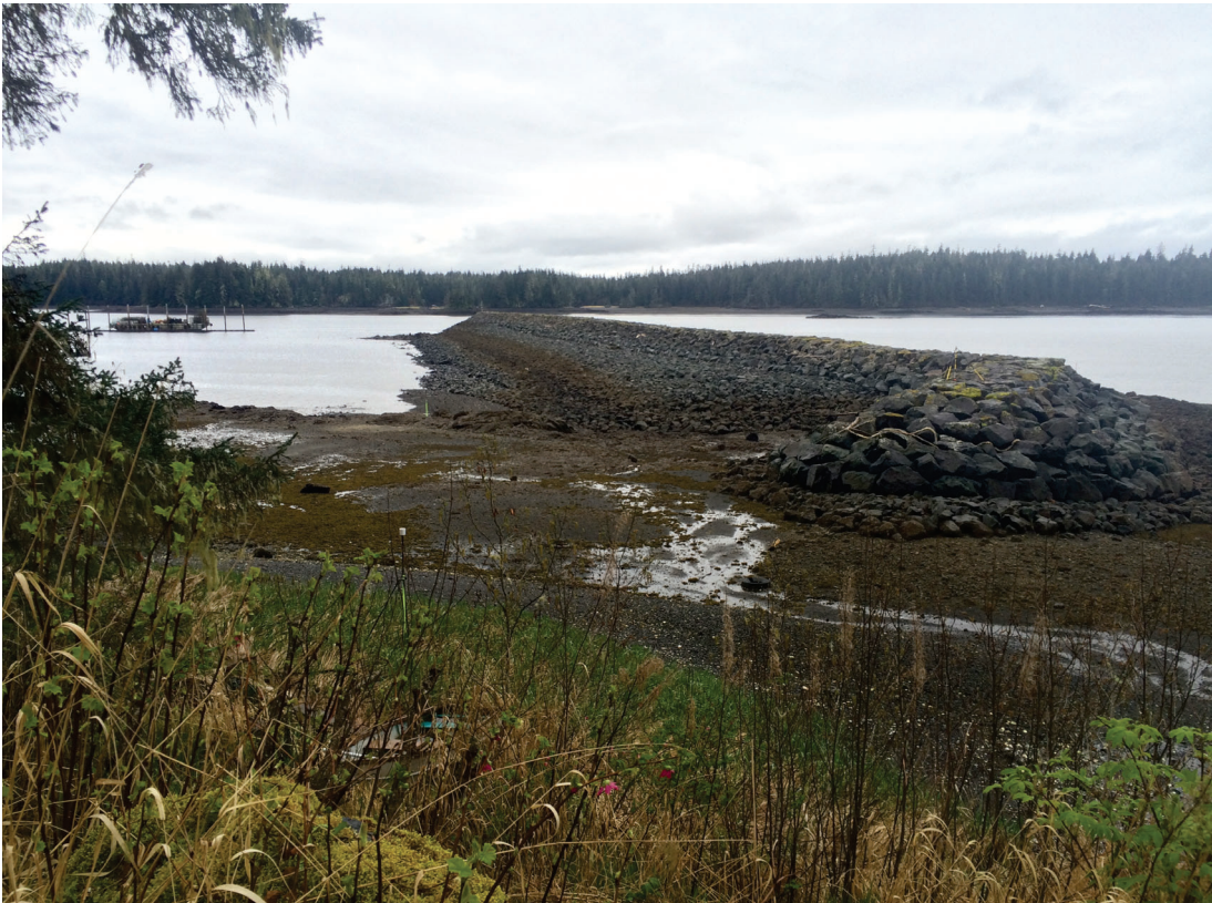
Kake Breakwater, April 2016
