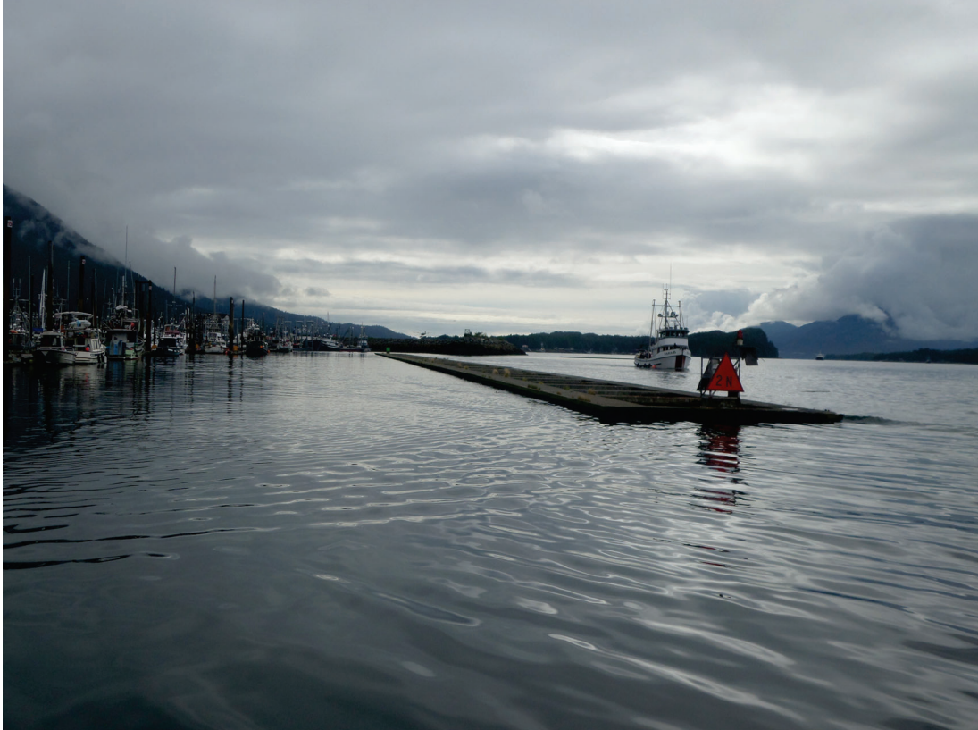
Large floating breakwater protecting the expanded harbor, August 2015
