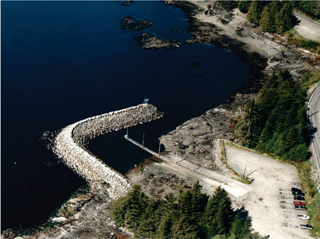
Southwest oblique of Mountain Point Breakwater, April 2005
