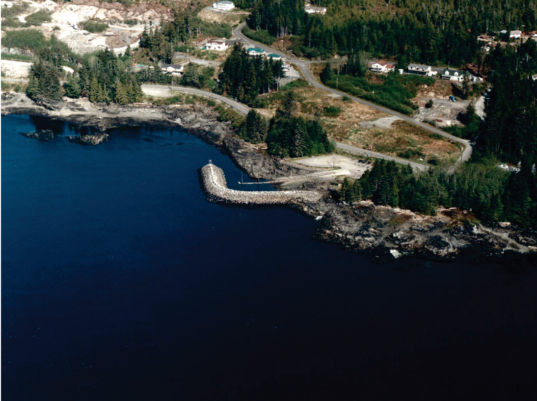
North oblique of Mountain Point Breakwater, April 2005
