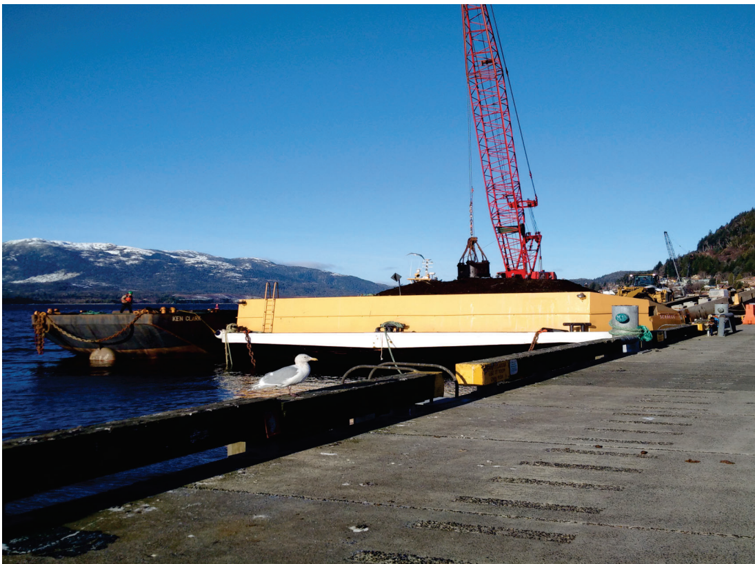
Transferring dredged material from scow to haul barges, February 2018
