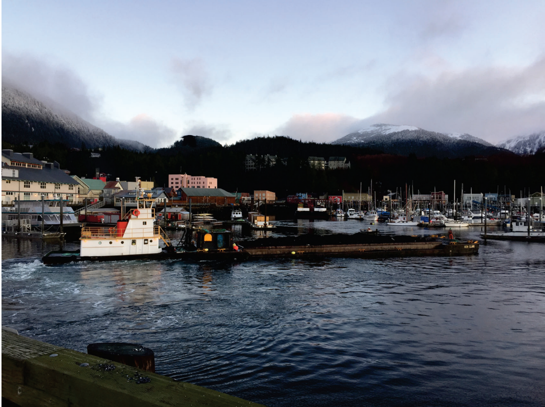
Moving dredged material for transfer to haul barges, February 2018
