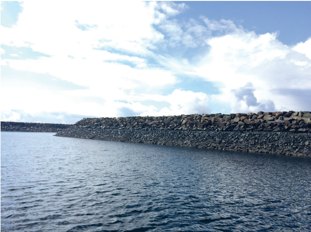
New Harbor Breakwater, May 2016
