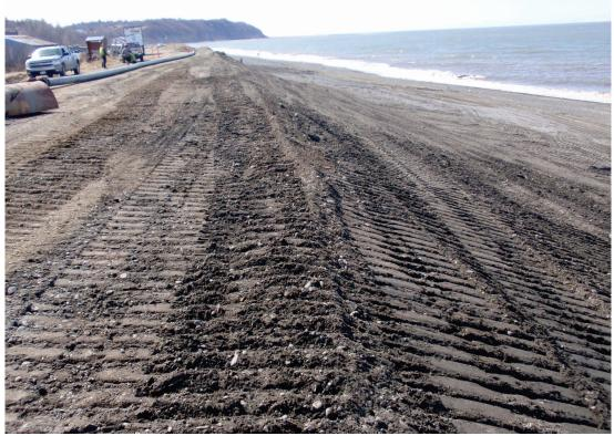
Leveling of dredged material over the revetment, May 2019
