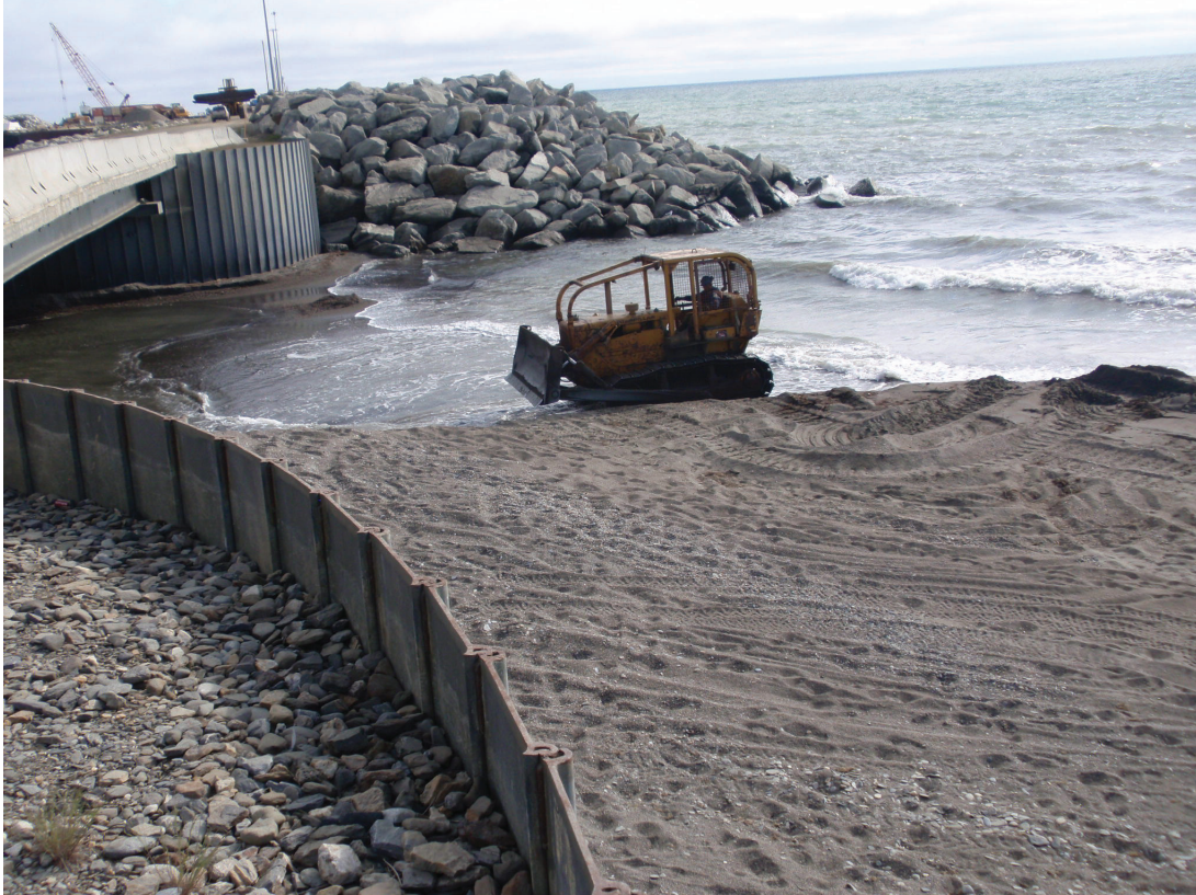
Pushing material under the causeway bridge towards the sediment trap, June 2019
