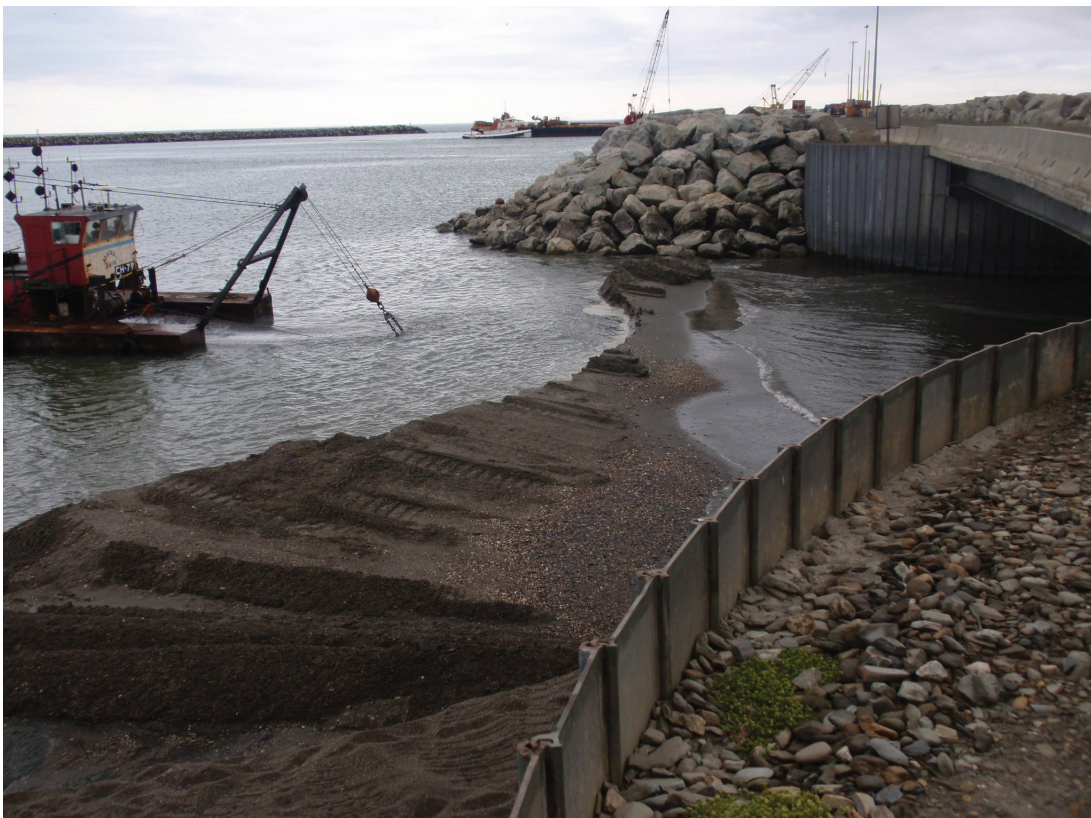
Dredging shoaled material near the sediment trap and causeway breach, June 2019
