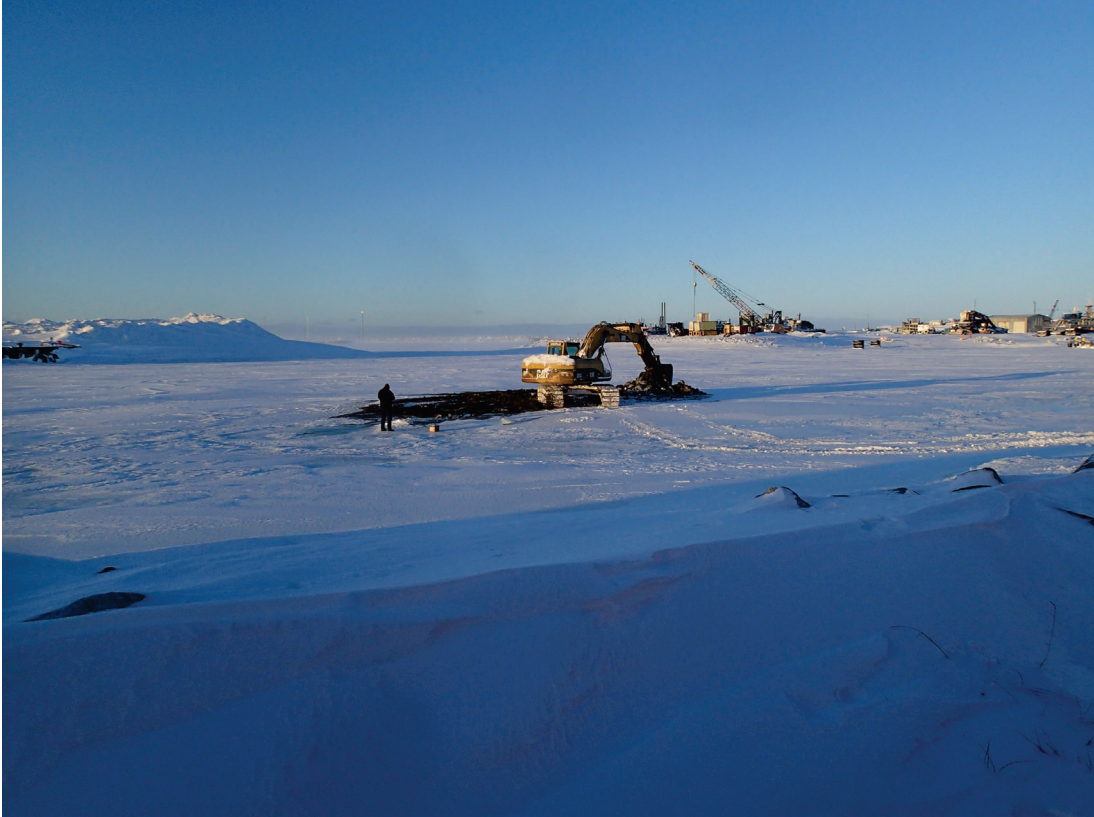
Geotechnical investigation for proposed widening of channel, February 2018
