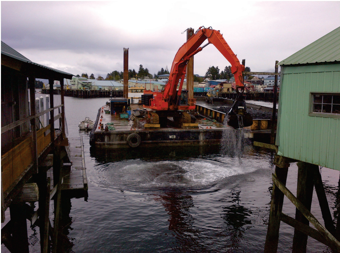
Dredging operations in Petersburg Harbor, 1 October 2013
