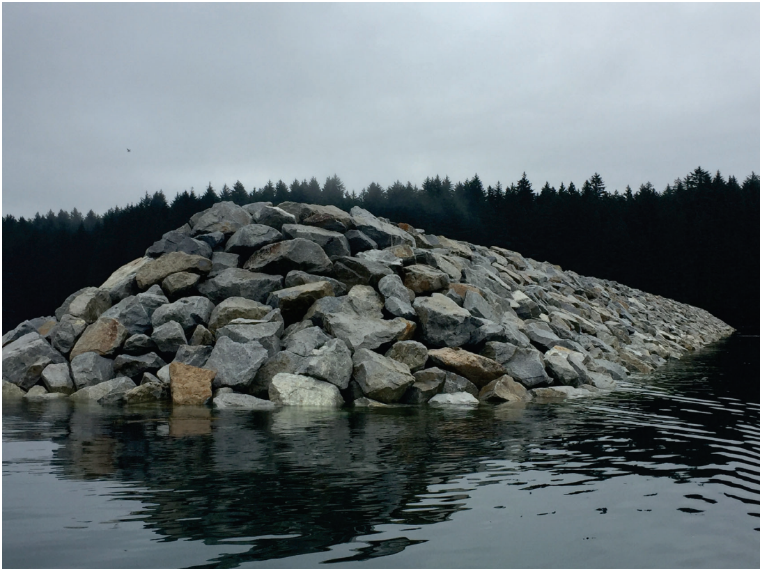
North End of New Breakwater, May 2018
