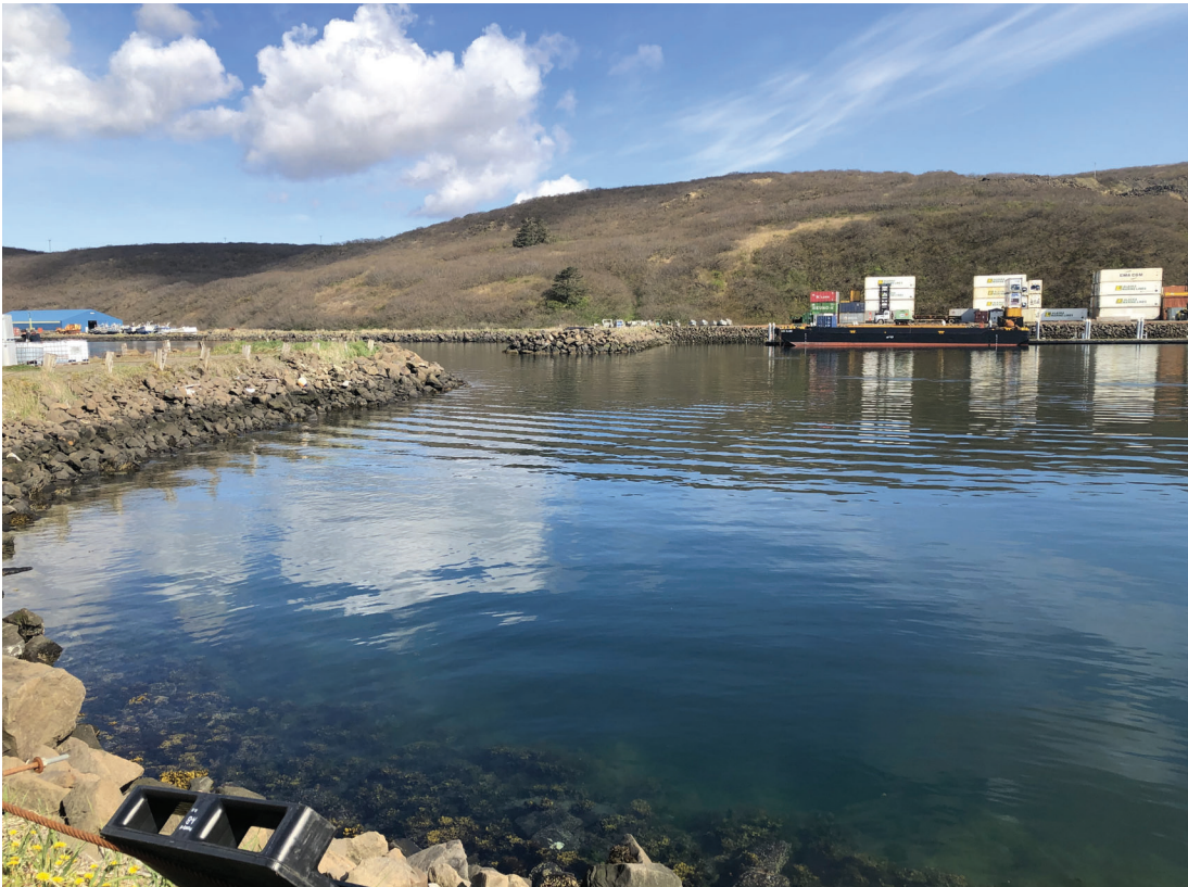
Sand Point New Harbor entrance channel, May 2019
