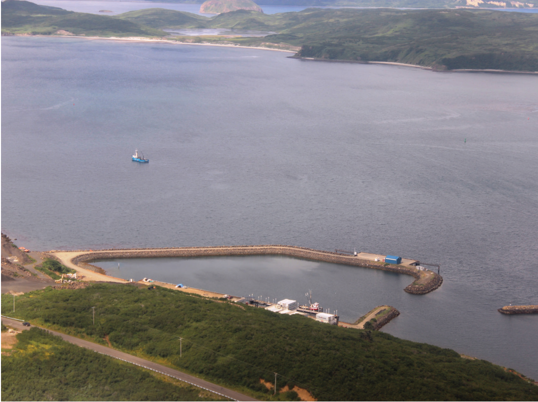
West oblique of Sand Point New Harbor, July 2014
