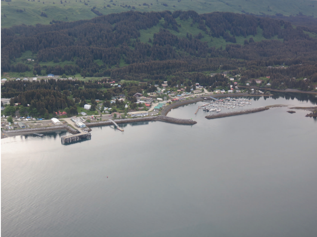
Northeast oblique of Seldovia Channel, August 2015
