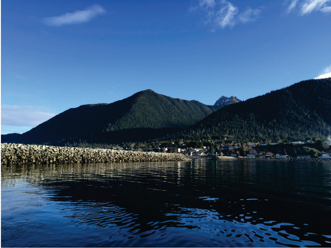
Channel Rock (Thomsen) Harbor Breakwater, March 2016
