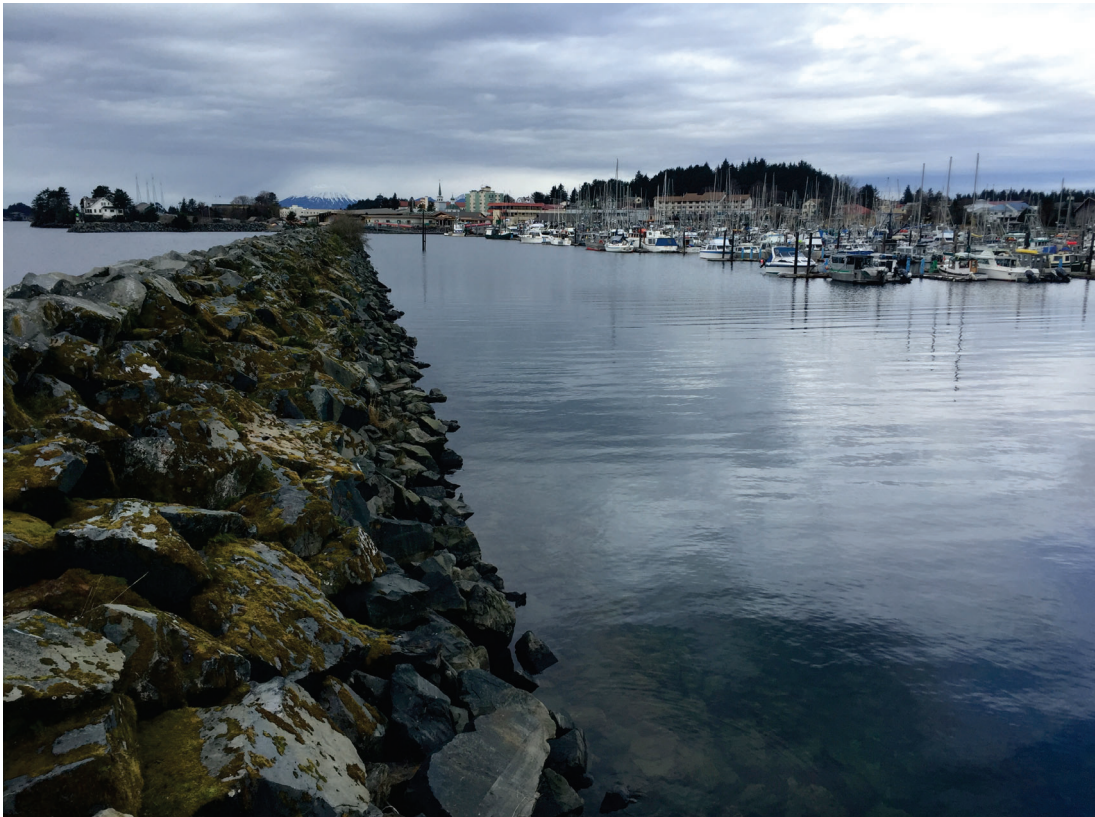
Crescent Bay Harbor and Breakwater, March 2016
