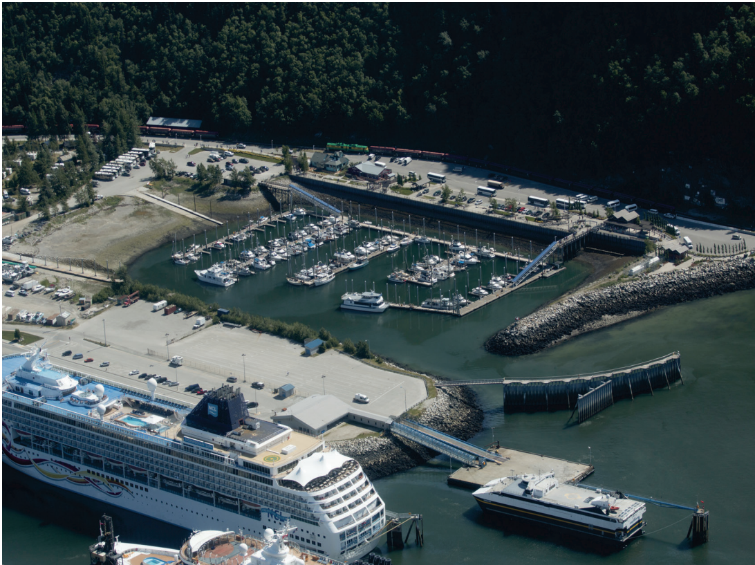
Northeast oblique of Skagway Harbor, 2016
