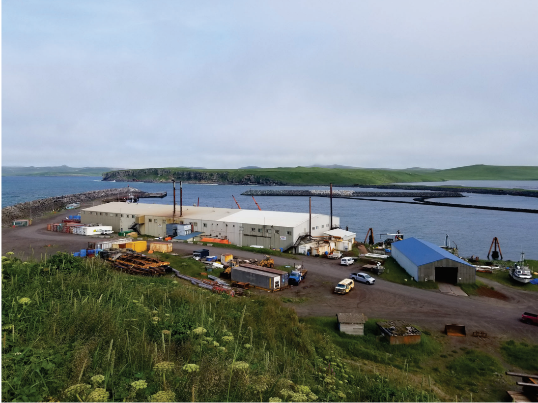
St. Paul Harbor Entrance Channel, July 2019
