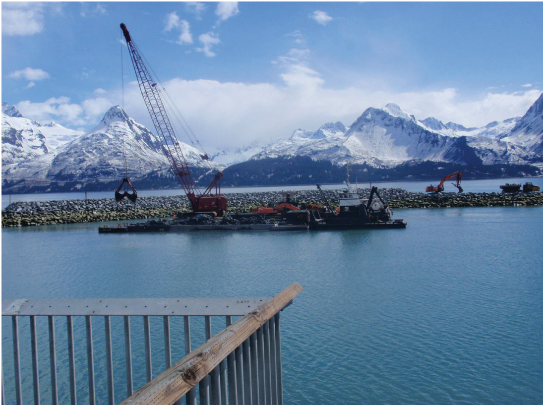
Final Dredging and Armor Rock Placement, May 2017
