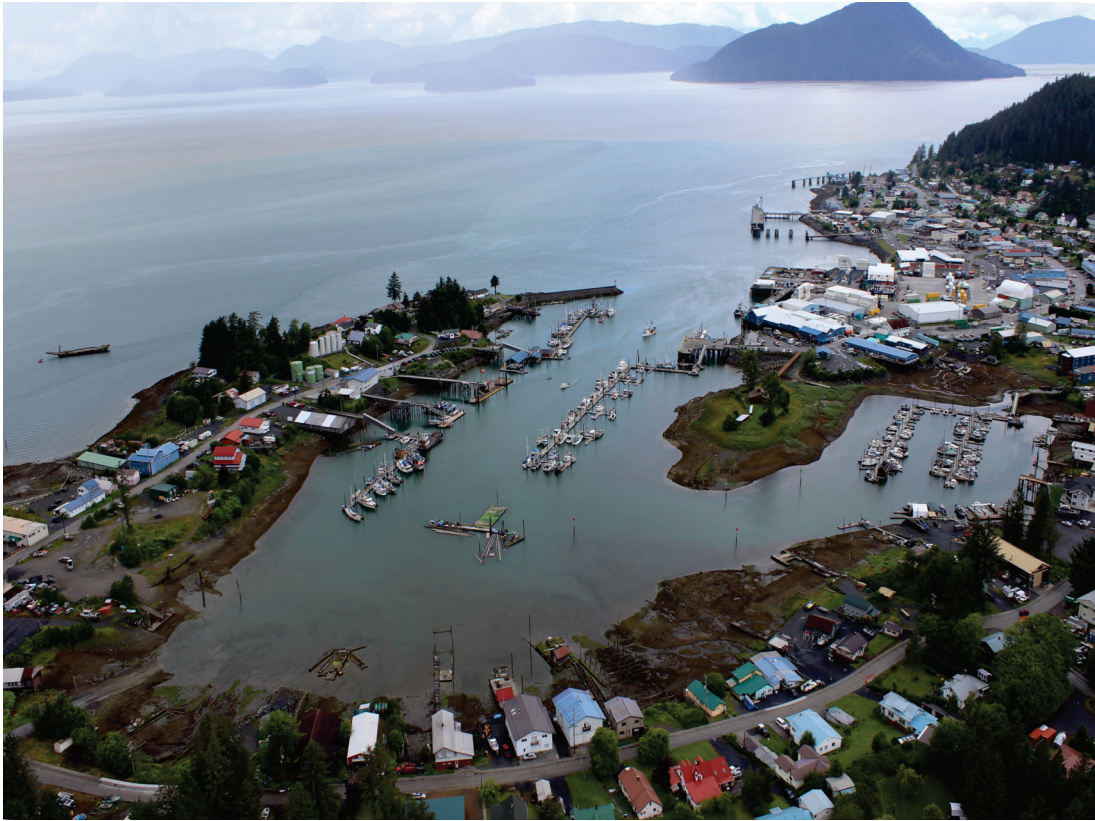
Oblique of Wrangell Harbor, July 2015.
