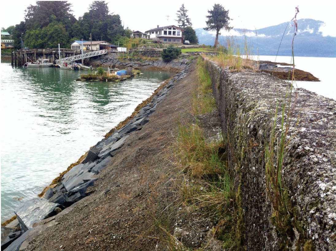
Wrangell Harbor Breakwater, July 2015.
