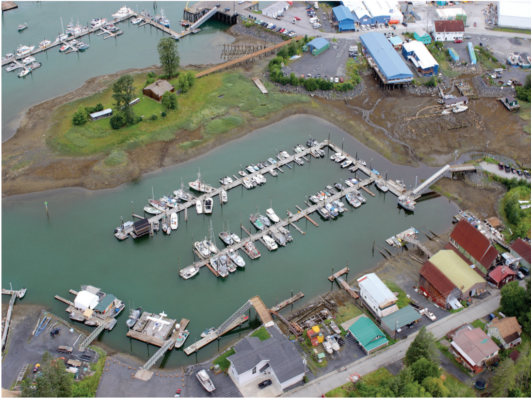
Oblique of Wrangell Harbor, July 2015
