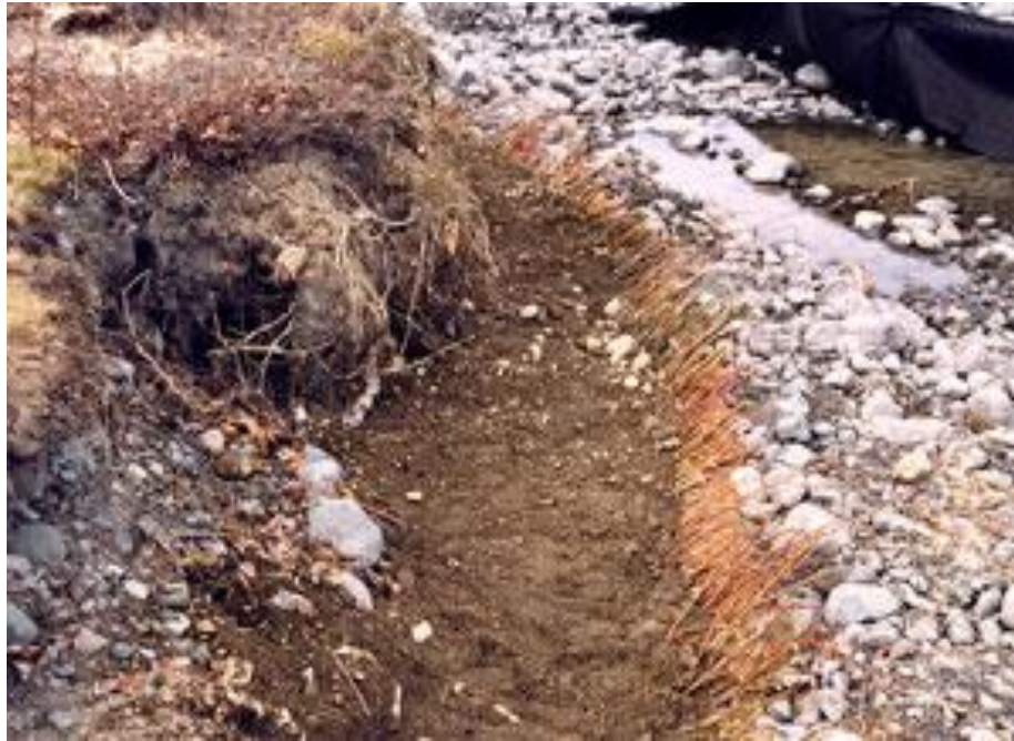
Photo 20: Live Siltation during Construction (ADF&G 2005)
