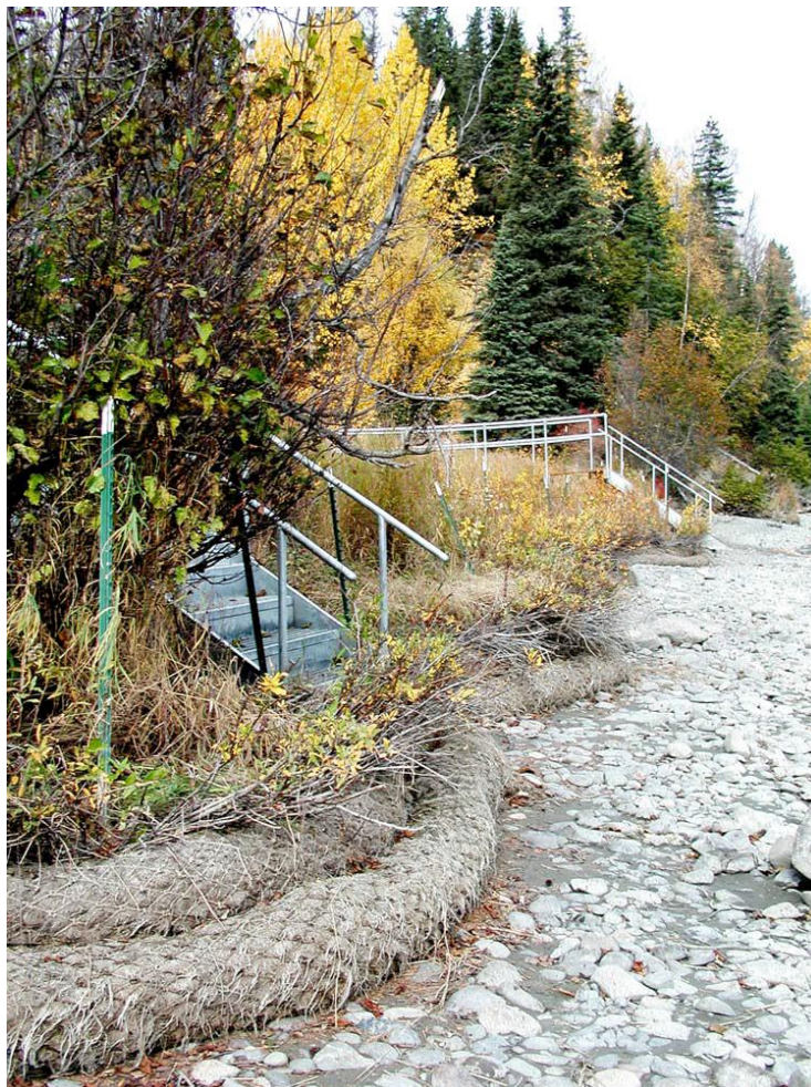
Photo 17: Coir Logs Installed at Slikok Creek (Weiner 2000)
