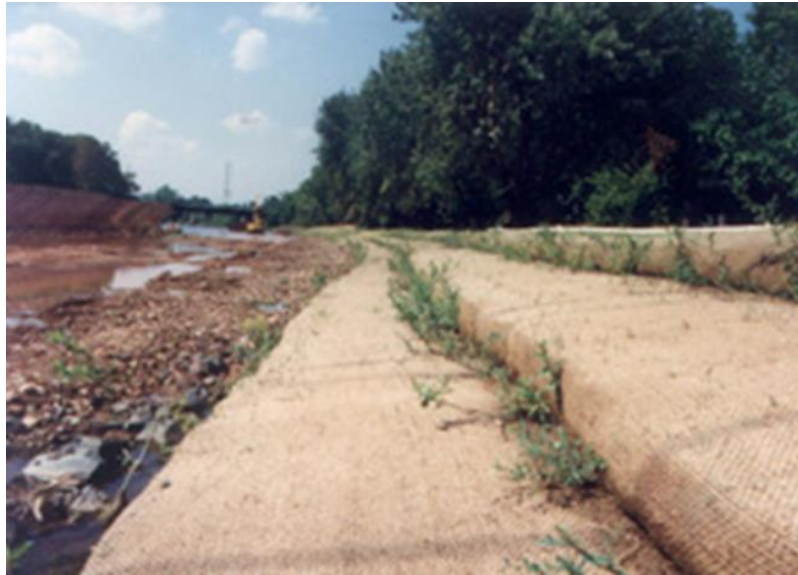
Photo 18: Coir Mat Lift Installation with Brush Layering
