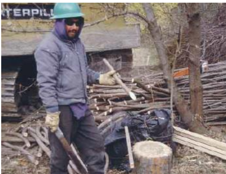
Photo 14: Preparing Dormant Cuttings for Live Stake Planting (Eubanks, C.E. and D. Meadows 2005)
