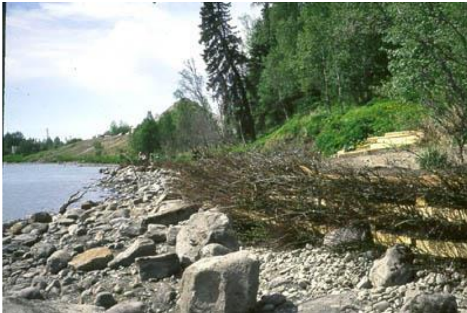
Photo 23: Vegetated Cribwall Installed along the Kenai River
