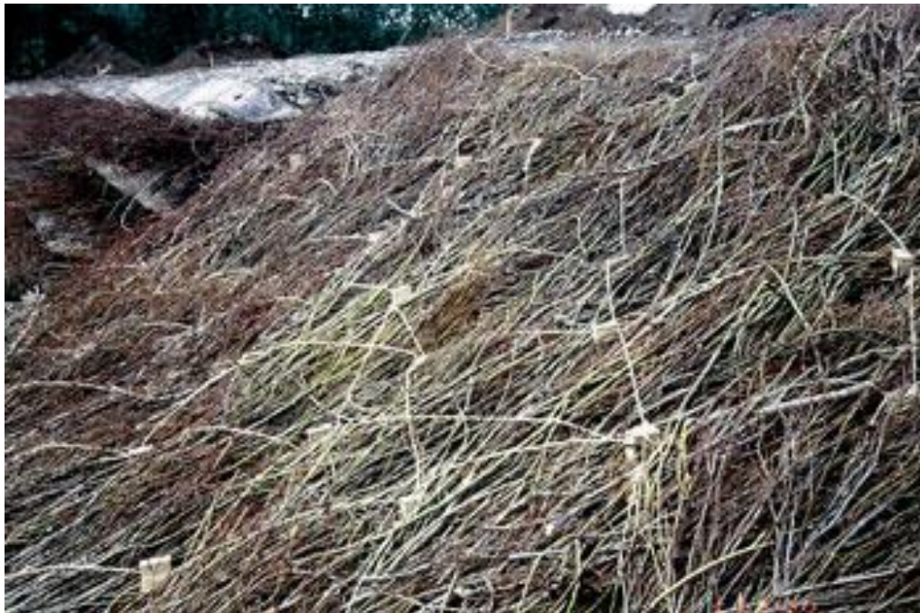
Photo 16: Brush Mattress Installation Secured with Jute Twine (ADFG 2005)
