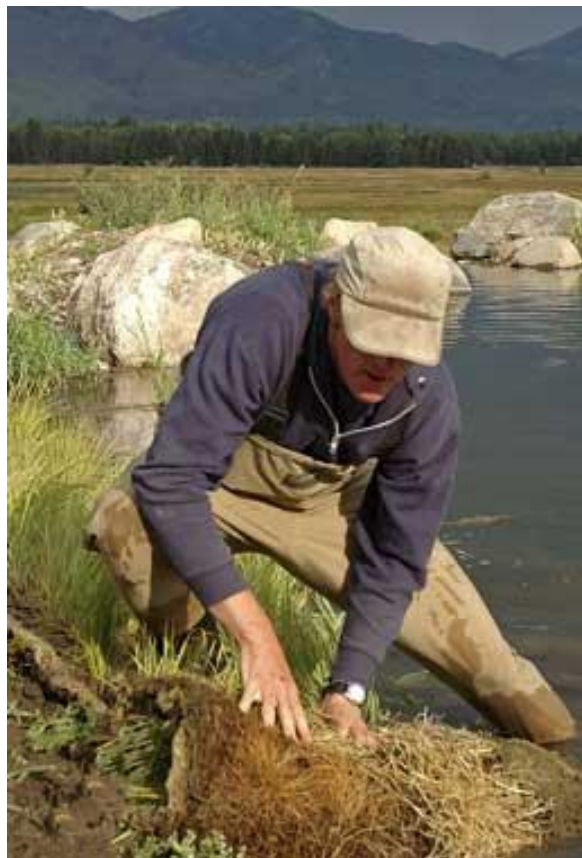
Photo 13: Placing Vegetative Mat as Restoration Treatment (North Fork Native Plants)
