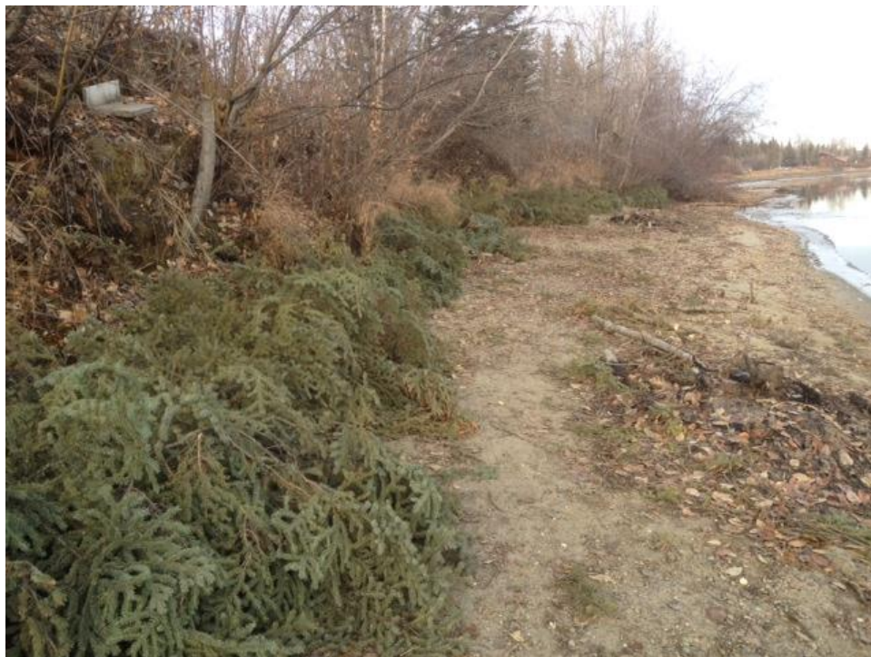
Photo 22: Spruce Tree Revetment on the Bank of the Chena River
