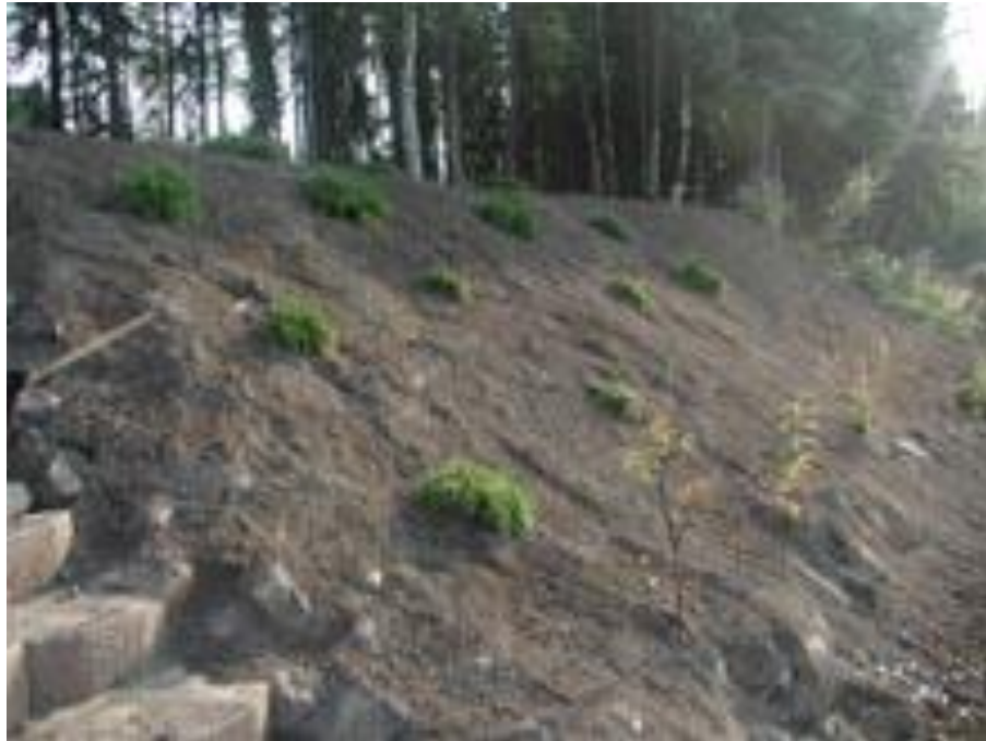
Photo 25: Vegetated Riprap with Willow Live Staking along the Chena River.
