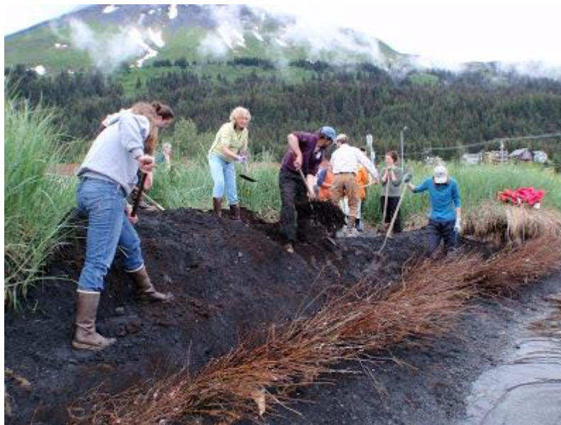
Photo 15: Brush Layering Installation at Scheffler Creek
