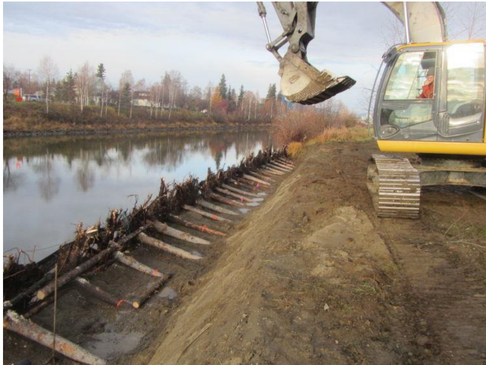
Photo 21: Root Wad Installation using Excavation and Trenching Method prior to Backfilling along the Chena River
