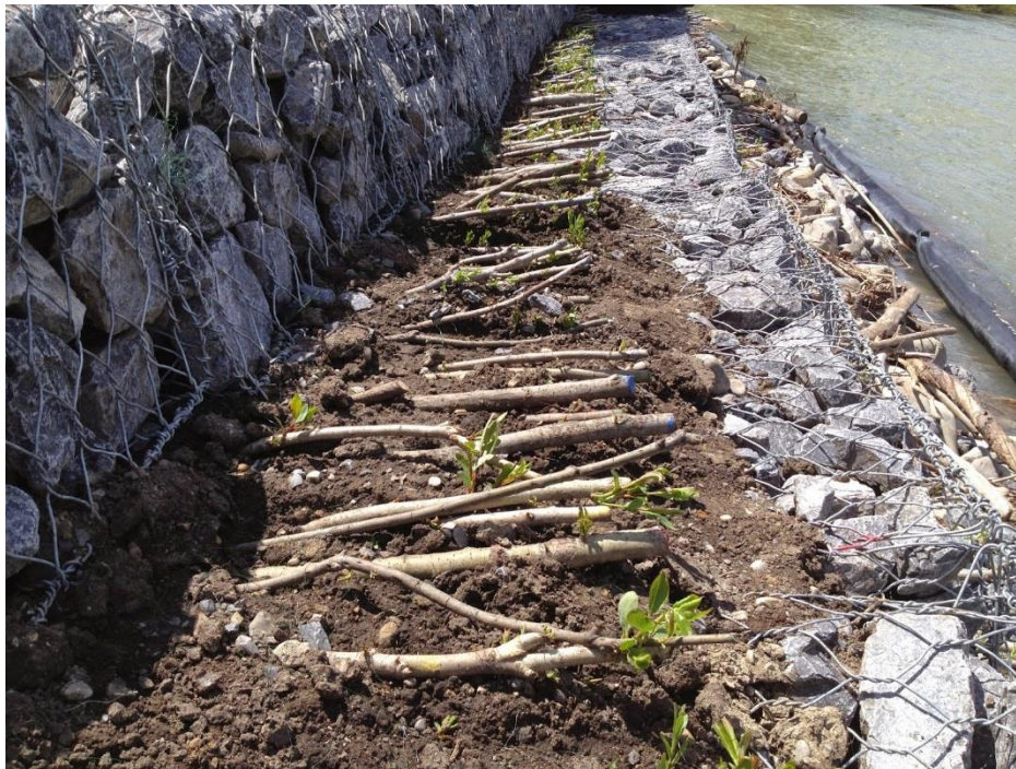
Photo 24: Dormant Cuttings Integrated into Gabion Construction
