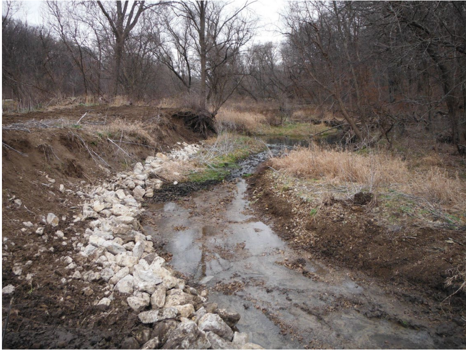
Figure 5: An example of toe slope stabilization. From ERDC's Streambank Erosion and Protection course (2022).
