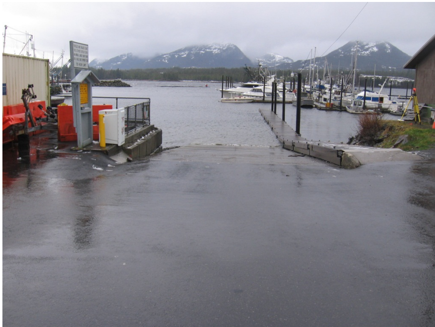
Figure 2 - Existing Single Lane Facility;
