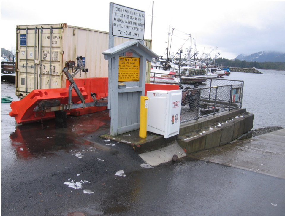
Figure 3 - MSE Retaining Wall, 'Kids Don't Float' Kiosk and Connex on left
