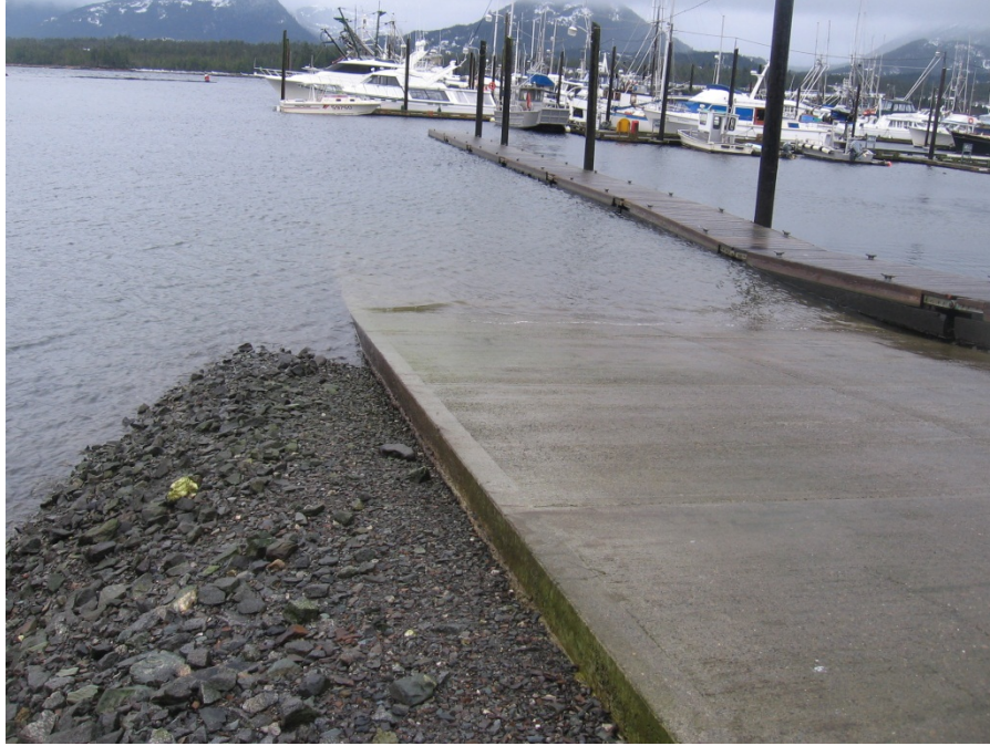
Figure 1- Existing Boat Launch Ramp, looking towards harbor from abutment
